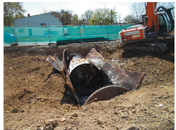
6: Removal of fuel tank in central site area, looking south-south-west
