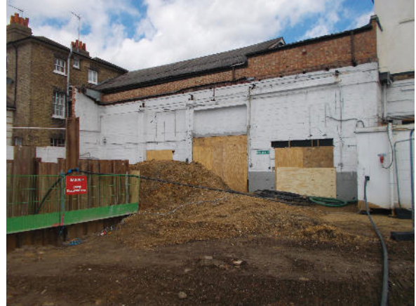
2: Western site area, looking north-west
