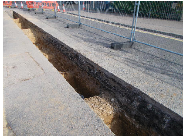
12: Service trench along North Road, looking north-west
