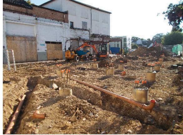
8: Piling and drainage trench in western site area, looking north-east
