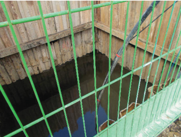
3: Drainage pit in western site area, looking north-west
