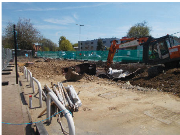
5: Removal of fuel tank in central site area, looking east-south-east
