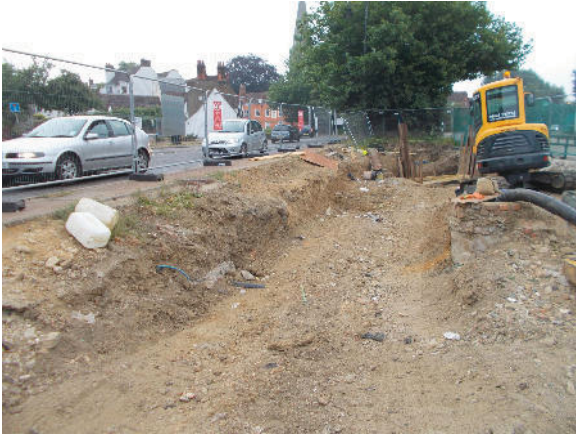
9: Ground reduction in eastern site area, looking east
