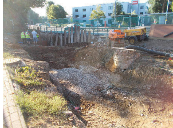
10: Additional ground reduction in eastern site area, looking south-east
