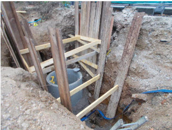
11: Excavation of the eastern site area, looking south-east
