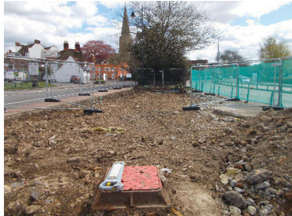
4: Ground reduction in eastern site area, looking east
