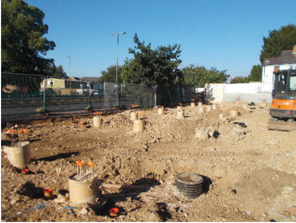
7: Piling in central/ western site area, looking south-west
