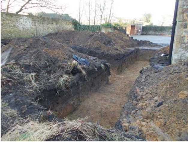
DP 7. Trench 2. Looking west.
