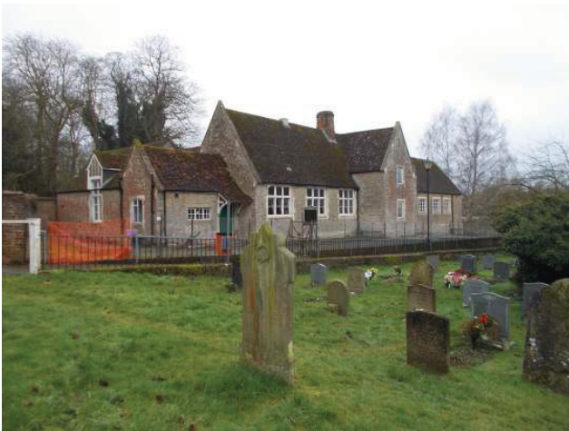
DP 1. Former Church Centre. Looking south-west.
