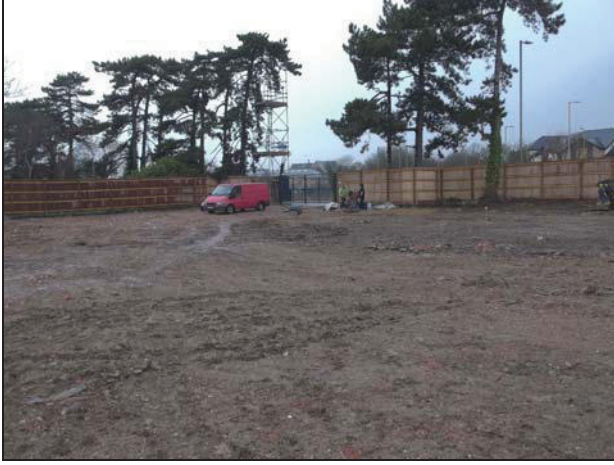
1 General view of the site before excavation
