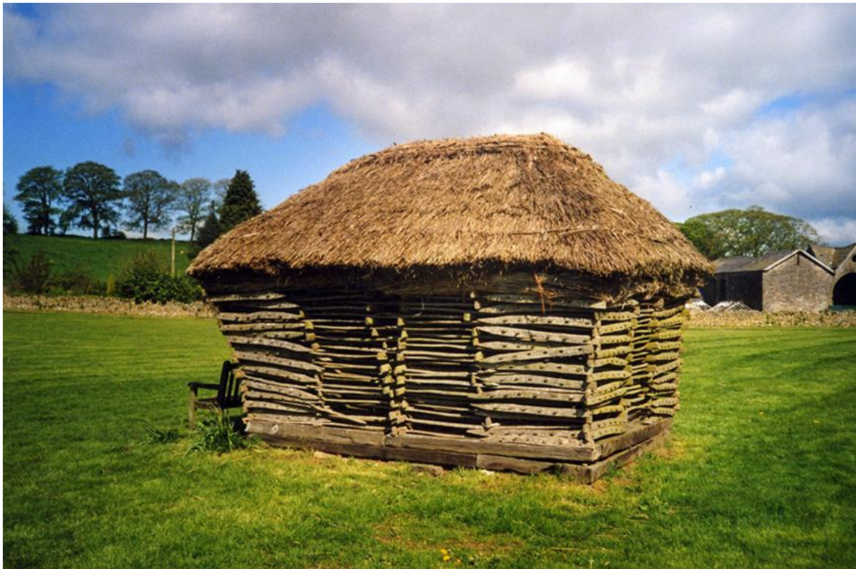
Plate 14: The Priddy hurdle stack; photograph by Graham E. Cook (g.e.cook@thatchinginfo.com); note the arrangement of beams supporting the base of the stack
