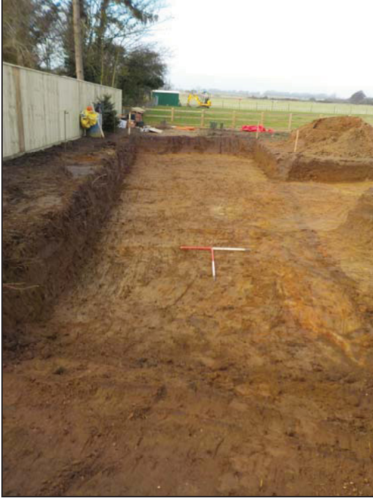
1 View of site looking north-west
