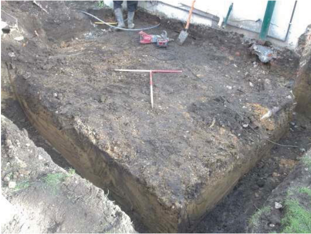
DP 7. Side extension. Foundation trenches and ground reduction. Looking east.
