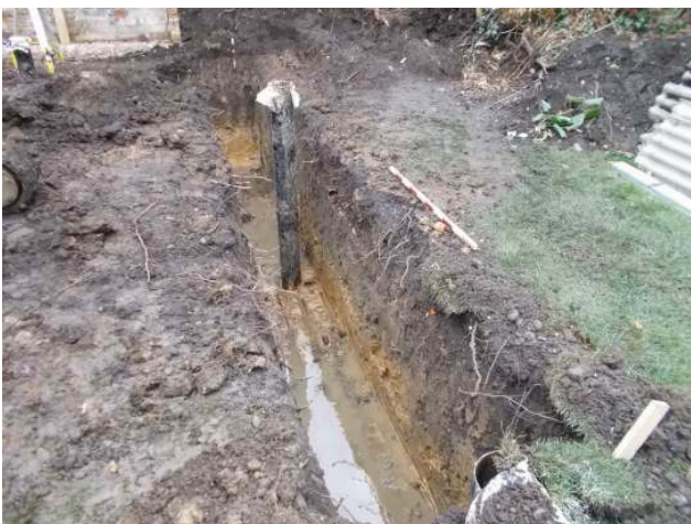
DP 5. Rear extension, south-west trench. Looking south-east.
