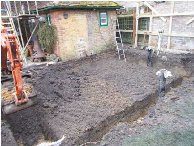
DP 3. Rear extension. Foundation trenches and ground reduction. Looking east.
