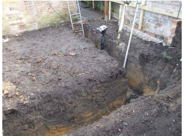
DP 2. Rear extension, foundation trenches. Looking east.
