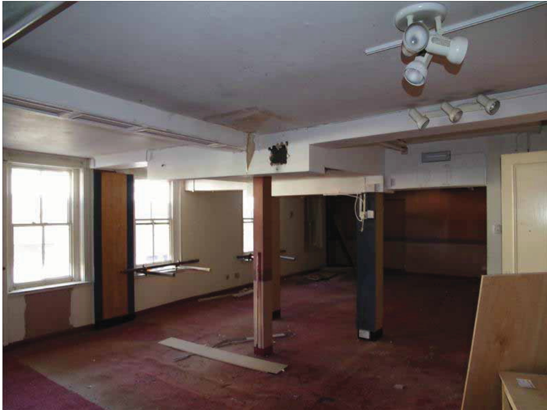
Plate 5 FF01, No. 17. Showing the 19 th century sash windows and the three columns replacing the original chimney stack. Taken from the north-west (DP 13)
