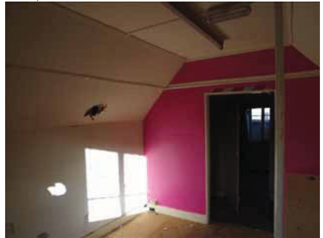
22 SF01, No. 15. Taken from the south-east.
