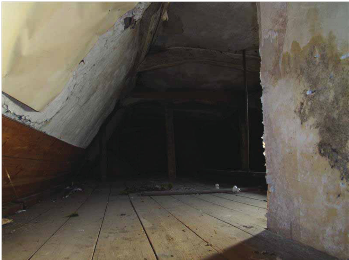
Plate 8 Roof structure above the main frontage of No. 15. Visible is the single truss with queen posts and cambered collars. Taken from the north (DP 25)
