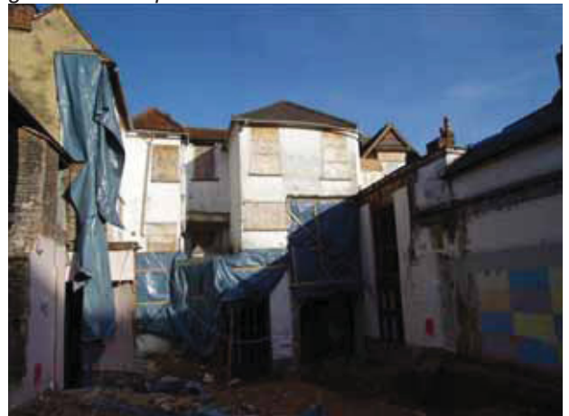
6 Rear elevation of No. 17. Taken from the west.
