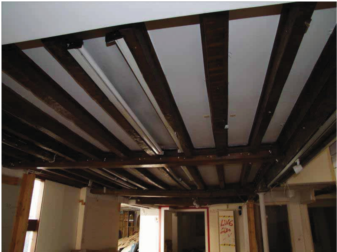
Plate 4 Roof timbers above ground floor of No. 15. (DP 11)
