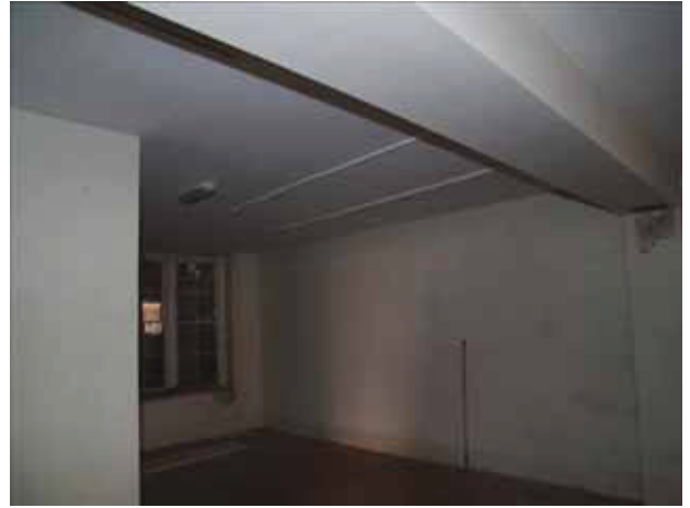
8 Interior ground floor space of No. 15. Taken from the north-west.
