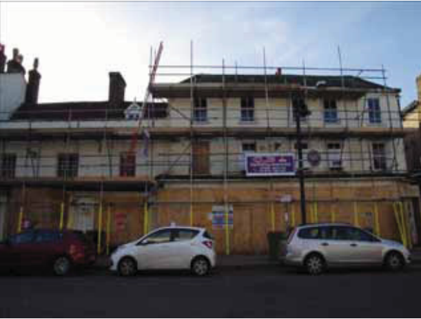
1 Main frontage of Nos. 15 & 17 North Street. Taken from the east.
