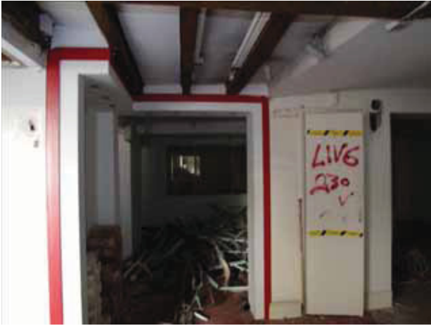
7 Interior ground floor space of No. 15. Taken from the west.
