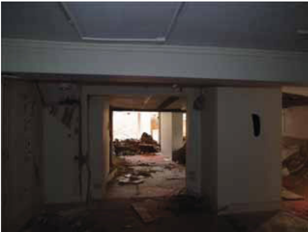
9 Interior ground floor space of No. 15. Taken from the east.
