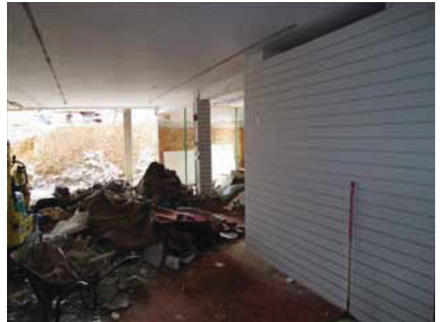
10 Interior ground floor space of No. 15. Taken from the south-east.
