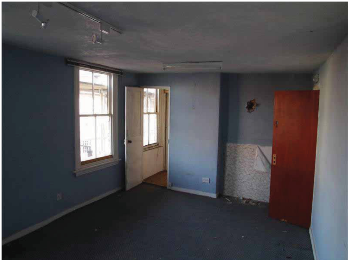
Plate 10 SF01, No. 17, showing sash windows with 1830s-1850s glazing bars, as well as preserved late 17 th /early 18 th century door, leading to SF1A (DP 32)
