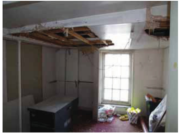
20 FF04, No. 15. Taken from the west.
