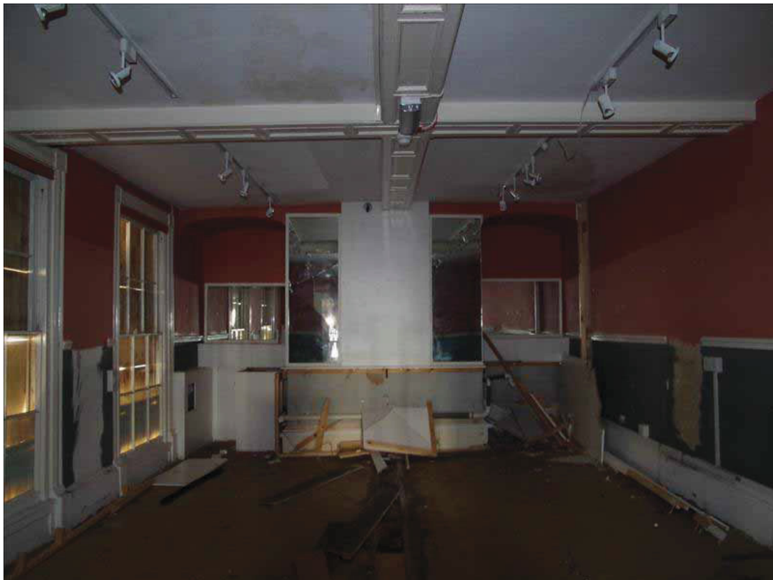
Plate 6 FF02, No. 17, showing chimney stack on the western wall, and two 19 th century sash windows on the southern wall. Taken from the east (DP 15).
