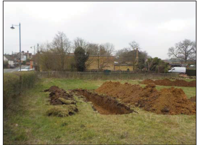
10 General view of site looking north
