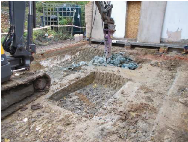
DP 3. New extension area. Removal of existing foundations. Looking west-north-west.
