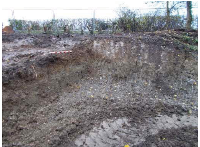
DP 4. New extension area. Looking south.
