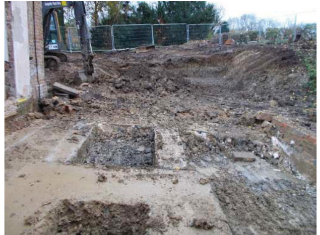
DP 2. New extension area. Looking south-east.
