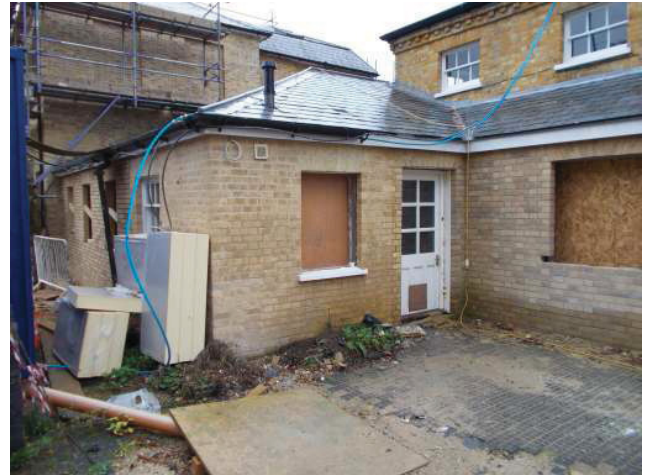
DP 8. New passage. Looking east.
