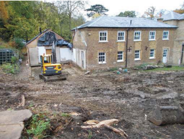
DP 1. Crowbury House with new extension area. Looking north.
