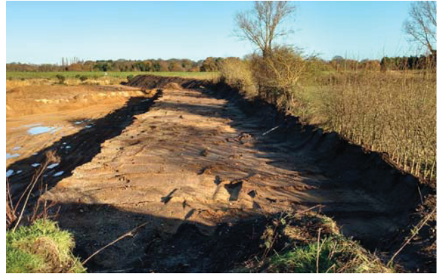
6 View of strip looking north-east
