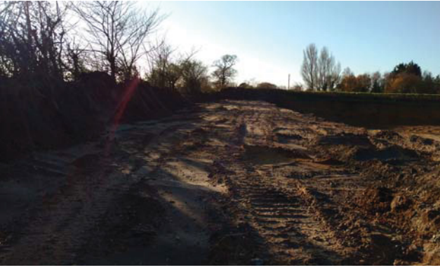
5 View of strip looking south-west
