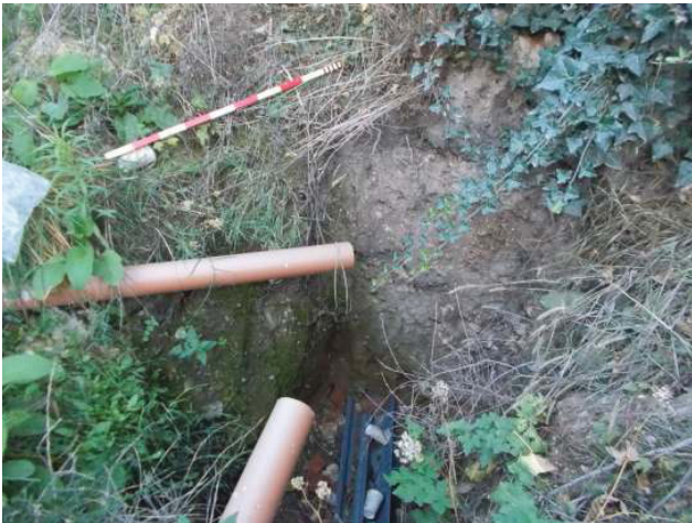
DP 9. North west soakway pit. Looking west.
