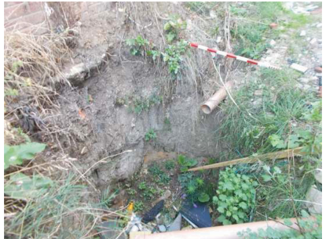
DP 10. South-west soakway pit. Looking north.
