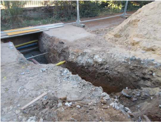
DP 7. Service trench. Looking south.
