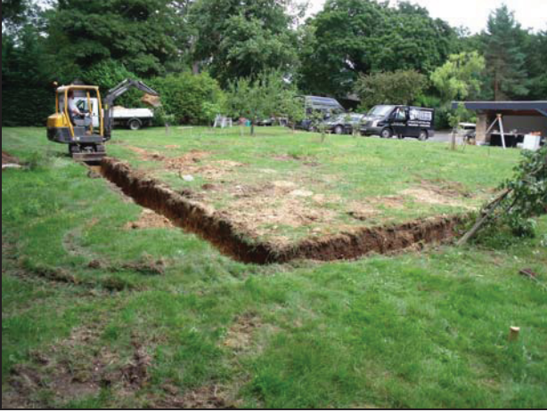
1 View of excavation area looking south-east
