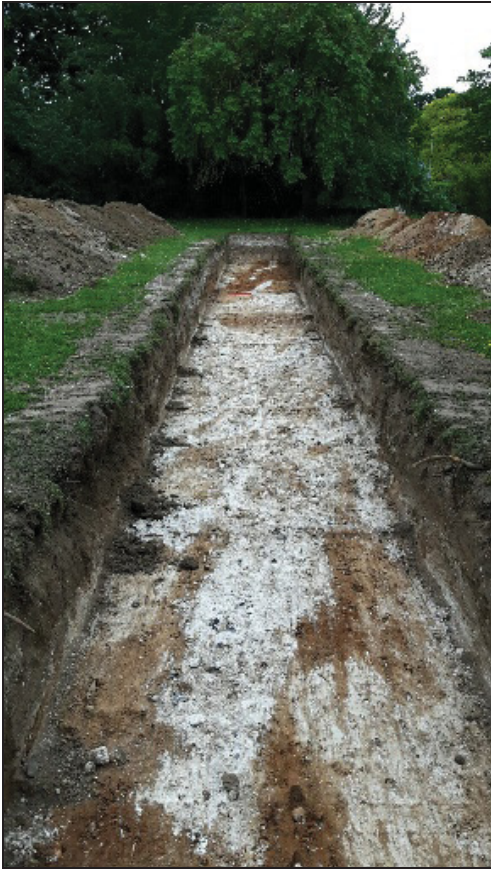
5 View of Trench 5 looking south-east
