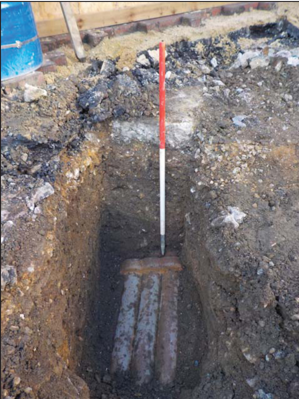
20 Test Pit 2 excavated during monitoring of groundworks
