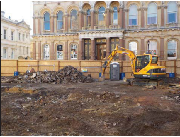
18 Monitoring of groundworks looking south-west
