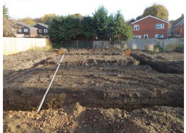
DP 8. Foundation trenches for new houses. Looking north-east.
