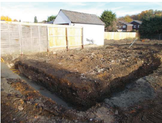
DP 11. Foundation trenches for new car port. Looking north.
