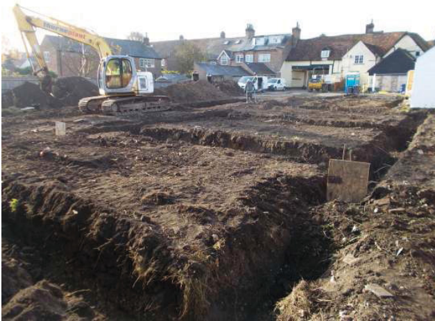
DP 7. Foundation trenches for new houses. Looking south-south-west.
