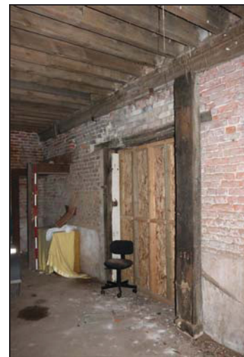
DP 60 North-west wall of the southern unit (Building 1: barn) showing doorway at the southern end infilled with modern boarding, taken from the north-east
