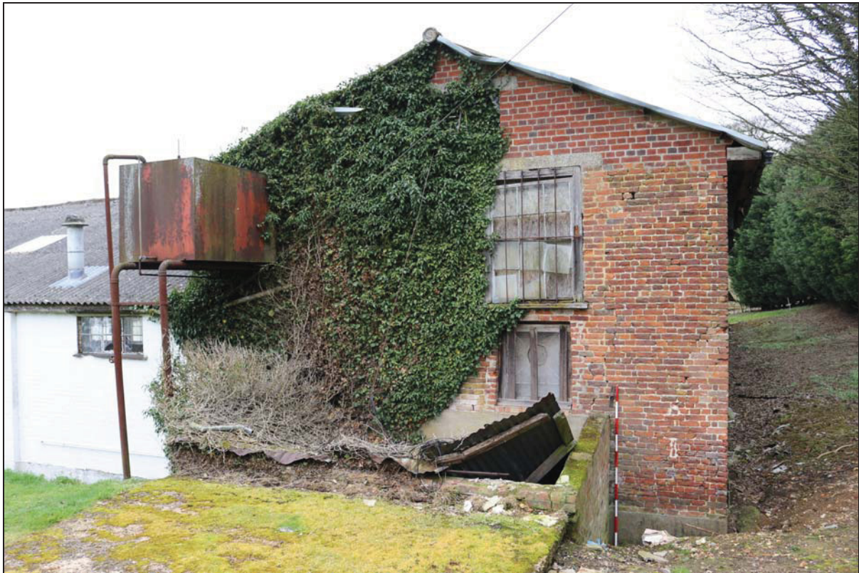
Plate 3 South-west elevation of the barn (Building 1), taken from the south-west (DP 11)
