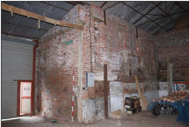
DP 31 South-west wall of the northern unit (Building 1: barn) showing blocked doorway, taken from the north-east
