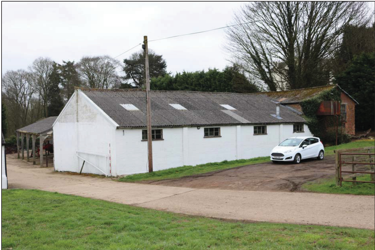
Plate 13 View of Building 2, taken from the west (DP 15)
