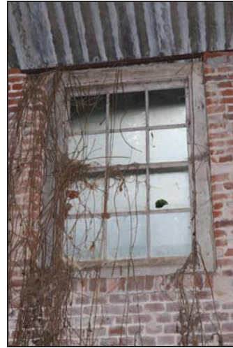
DP 38 Detail of the high-set six-over-six sash window on the south-east wall of the northern unit (Building 1: barn), taken from the north-west
