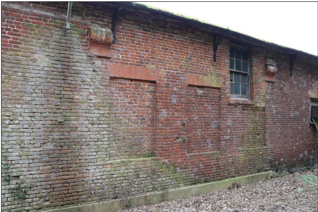
Plate 4 Detail of the south-east elevation (Building 1: barn) showing central set of blind panels framed by corbels, taken from the south (DP 79)
