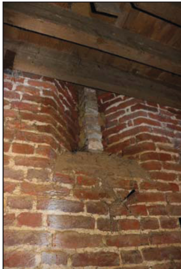
DP 57 South-west wall of the southern unit (Building 1: barn) showing infilled wind-eye, taken from the north-east
