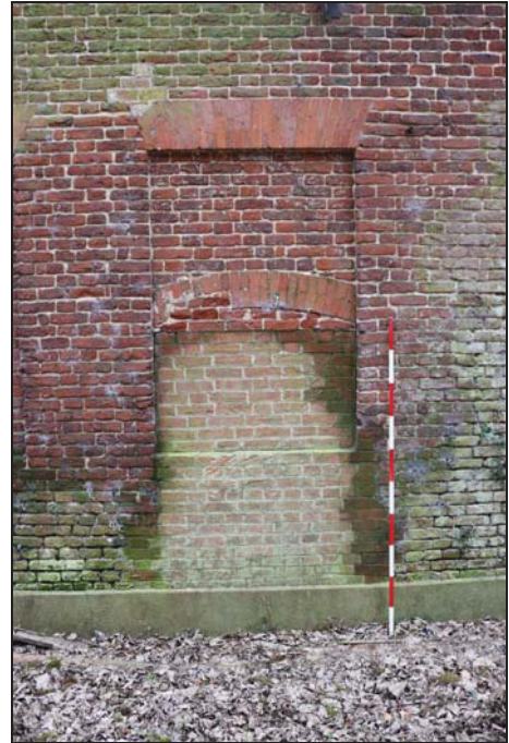
South-east elevation (Building 1: barn) showing blind panel with inserted aperture subsequently blocked, taken from the south-east
