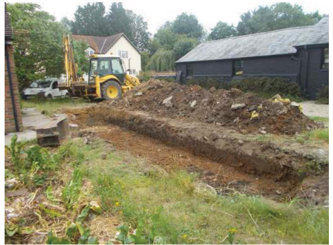
DP 2. Trench 1. Looking west.
