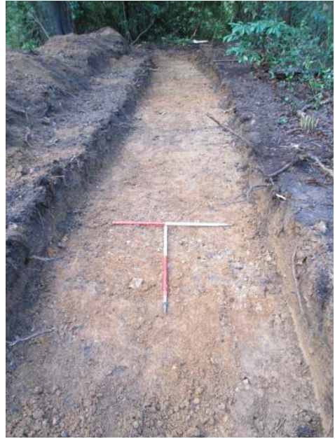
DP 8. Trench 2. Looking south-east.
