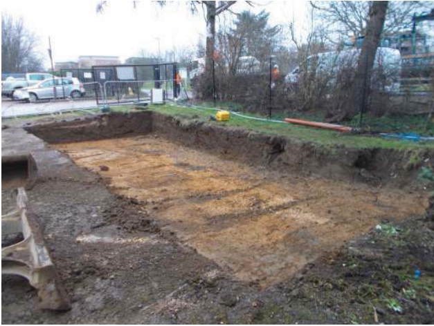
DP 7. Excavation for new pumping station. Looking north-north-east.
