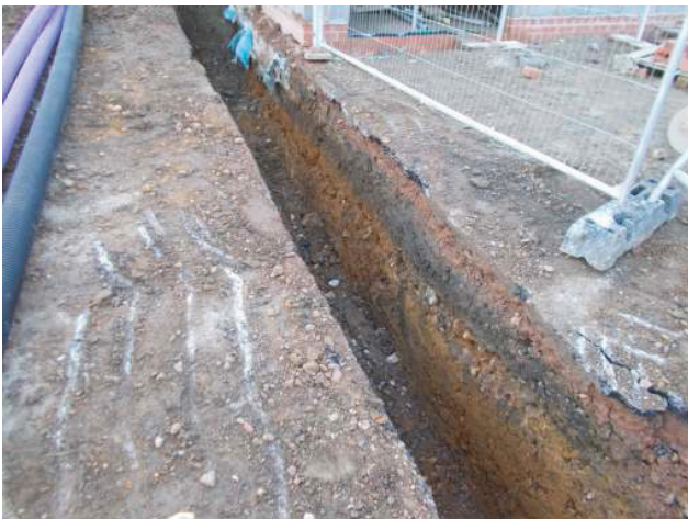
DP 11. Service trench for new pumping station. Looking east.
