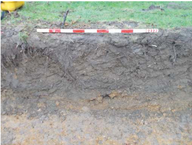
DP 9. Excavation for new pumping station. Sample section 3. Looking east-north-east.
