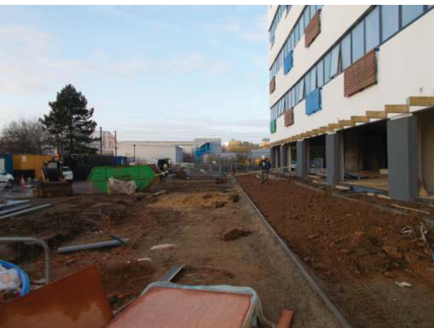
DP 5. Works to the south of the building. Looking west-south-west.
