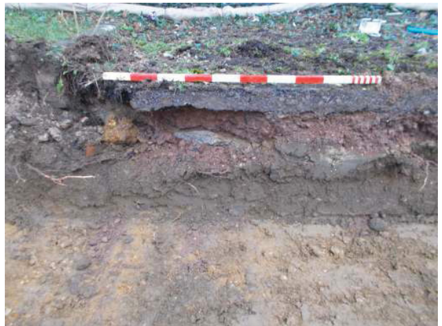
DP 10. Excavation for new pumping station. Sample section 4. Looking west-south-west.
