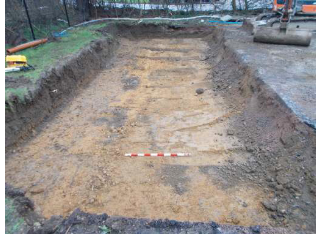
DP 8. Excavation for new pumping station. Looking south-south-east.
