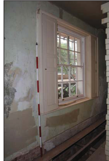
DP 64 Sash window with shutters on the west side of Room GF02, taken from the south-east
