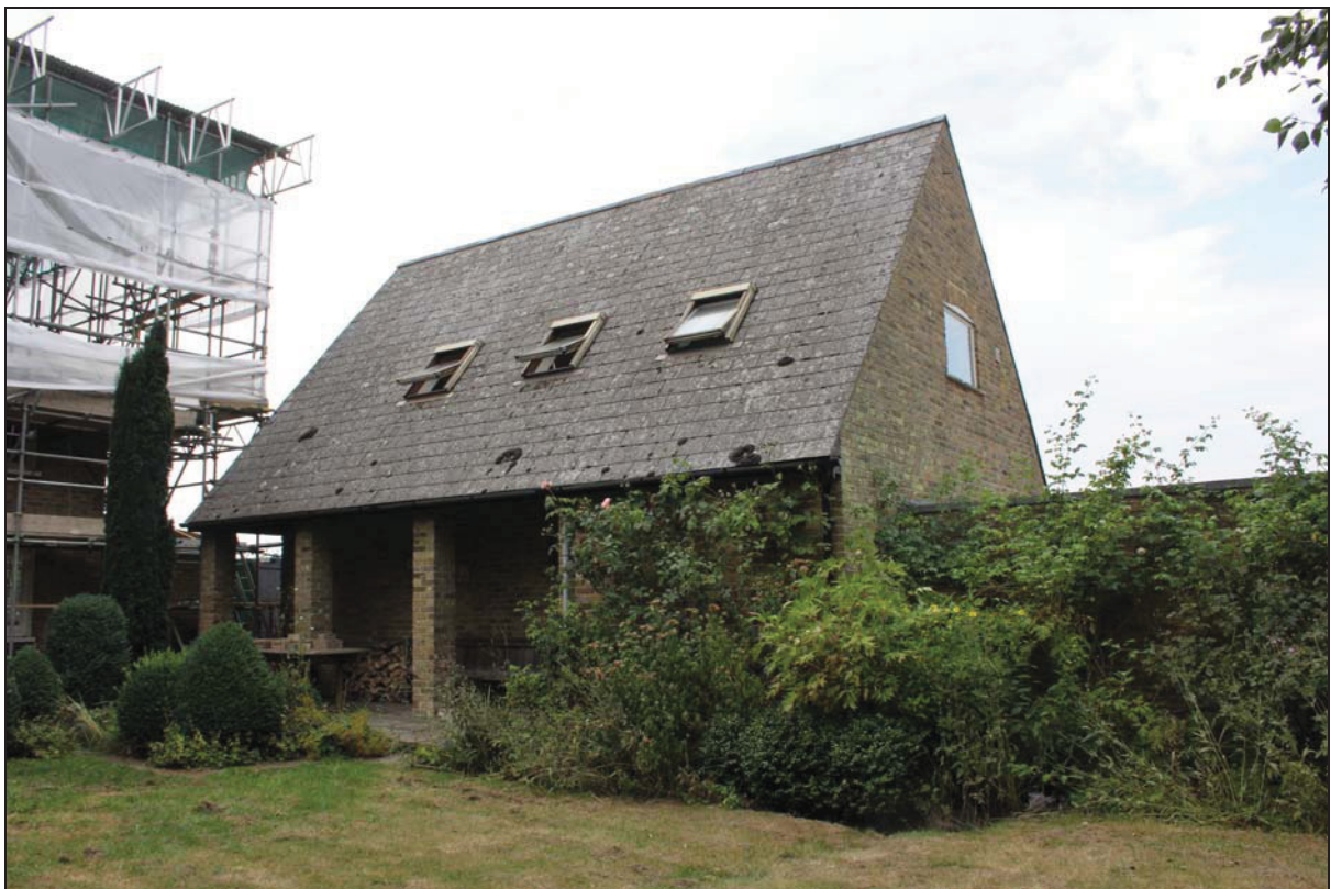
Plate 20 South side of the modern outbuilding, taken from the south (DP45)
