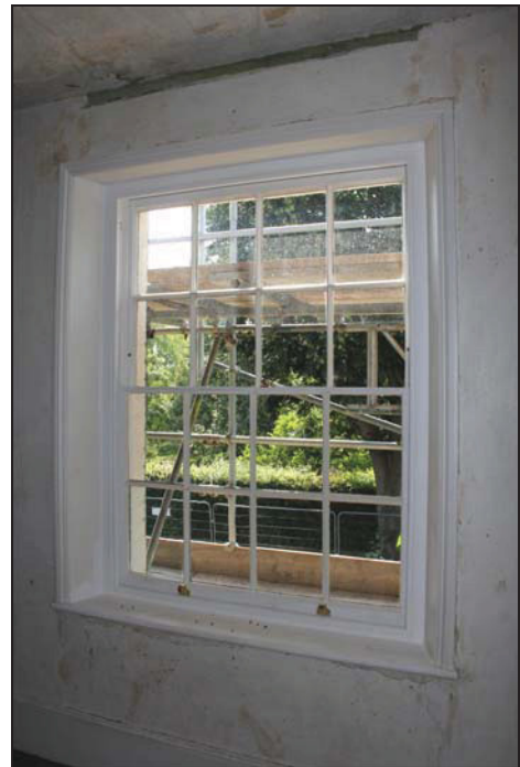
Slender moulded glazing bars on the sash window on the east side of Room FF05, taken from the west
