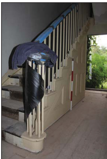
DP 53 View of the staircase (GF01), taken from the south-west
