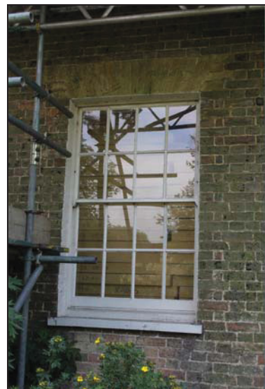
DP 36 Recessed sash window on the east elevation with a flat gauged brick arch, taken from the east
