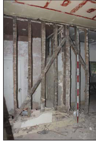
DP 2 Primary-braced studwork partition in Room GF05 after removal of lath and plasterwork, taken from the north-east
