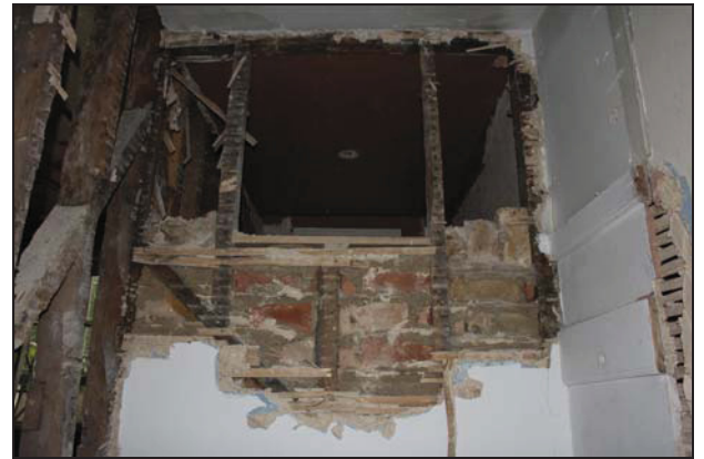
DP 2 Primary-braced studwork partition in Room GF05 after removal of lath and plasterwork, taken from the north-east
