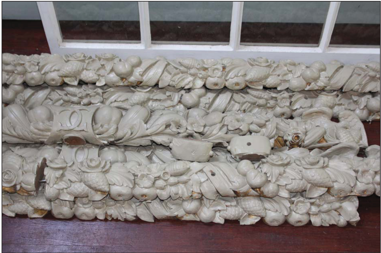
Plate 6 Decorative cornice formerly installed in Room GF02 stored prior to reinstallation (DP106)
