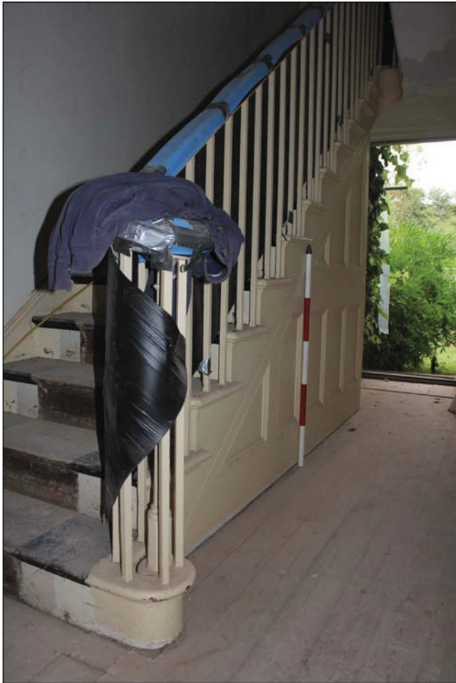
Plate 5 View of the staircase (GF01), taken from the south-west (DP53)
