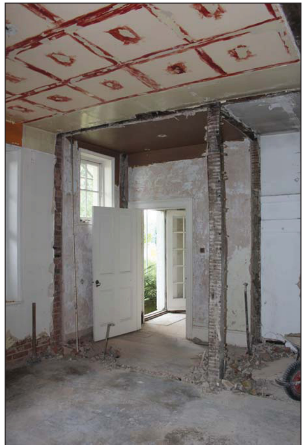
Plate 12 Room GF05 after removal of the primary-braced partition during the planned works, taken from the north-west (DP16)
