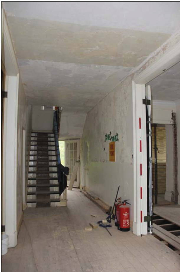
Plate 4 Entrance hall GF01, taken from the west (DP50)
