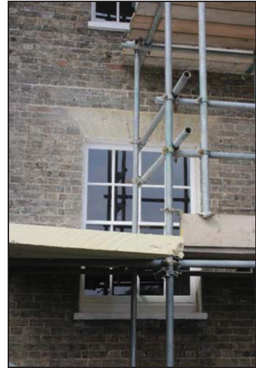
DP 32 Recessed sash window on the south elevation with a flat gauged brick arch, taken from the south
