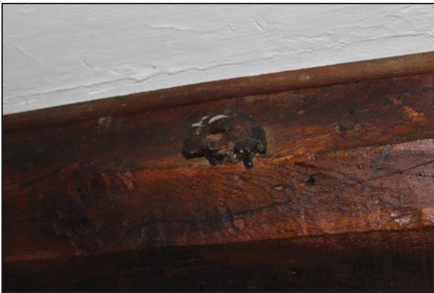
Mid-rail on the north-east side of Room GF01 showing redundant diamond mullion mortices, taken from the south-west
