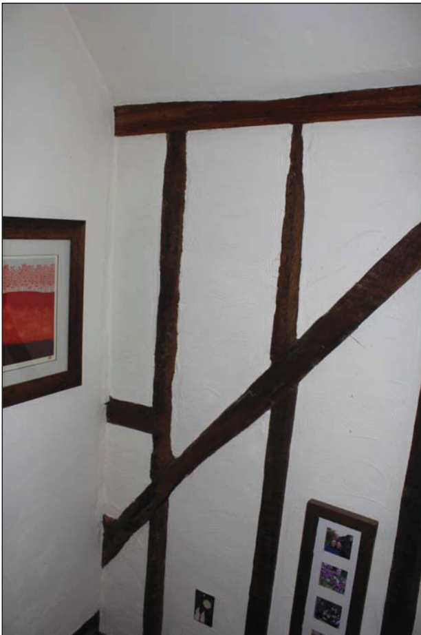
Plate 15 North-west wall of Room FF03 showing primary-braced studwork, taken from the south-east (DP 41)
