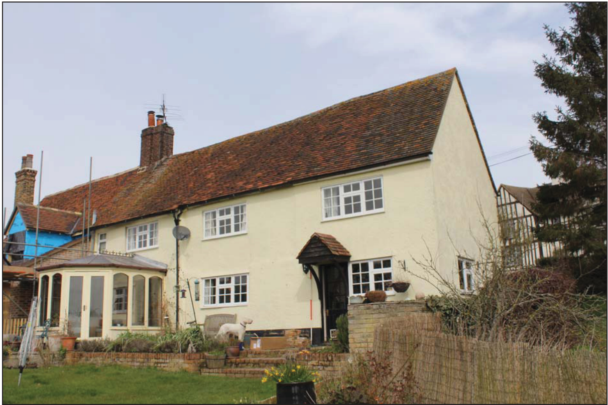
Plate 3 South-west elevation of Lordship Cottage, taken from the south-west (DP 02)
