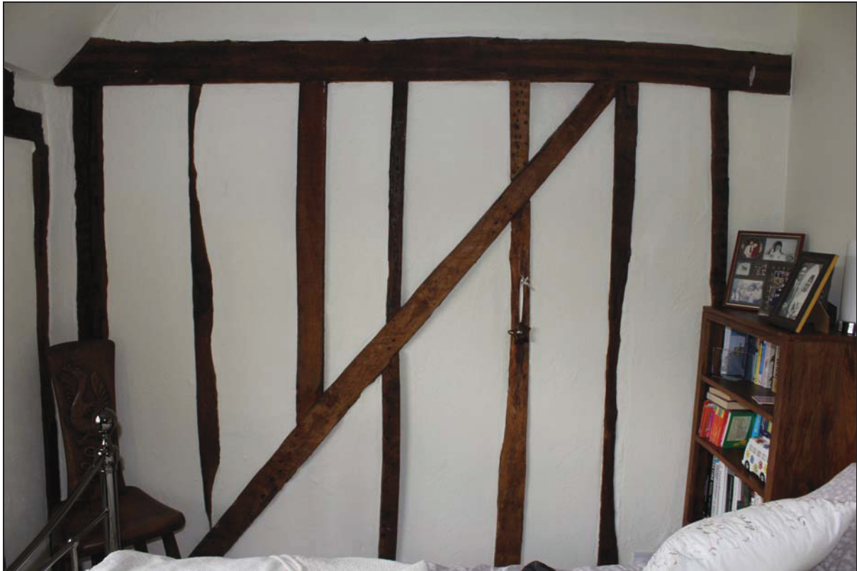
Plate 15 North-west wall of Room FF03 showing primary-braced studwork, taken from the south-east (DP 41)
