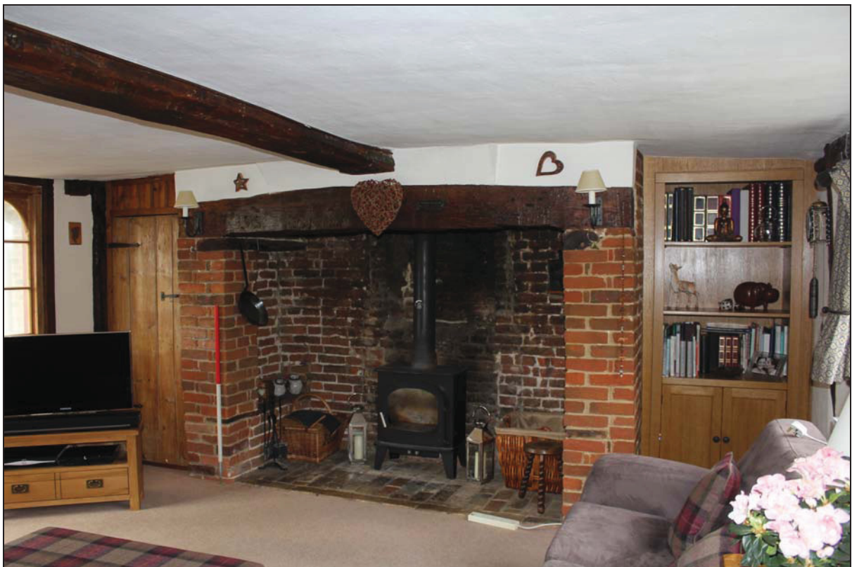
Plate 4 Inglenook fireplace in the historic core (GF01), taken from the south-east (DP 10)
