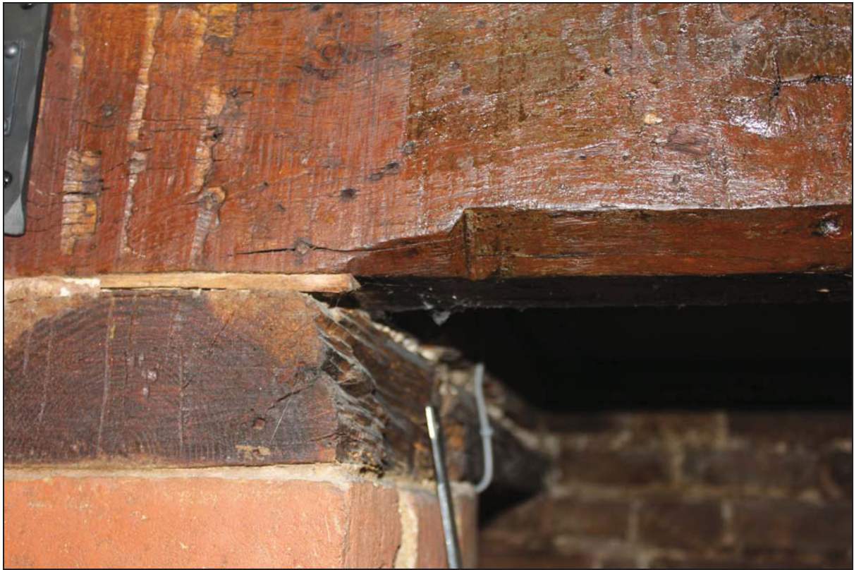
Plate 5 Lambs tongue chamfer stop on the fireplace bressummer in Room GF01, taken from the south-east (DP 11)
