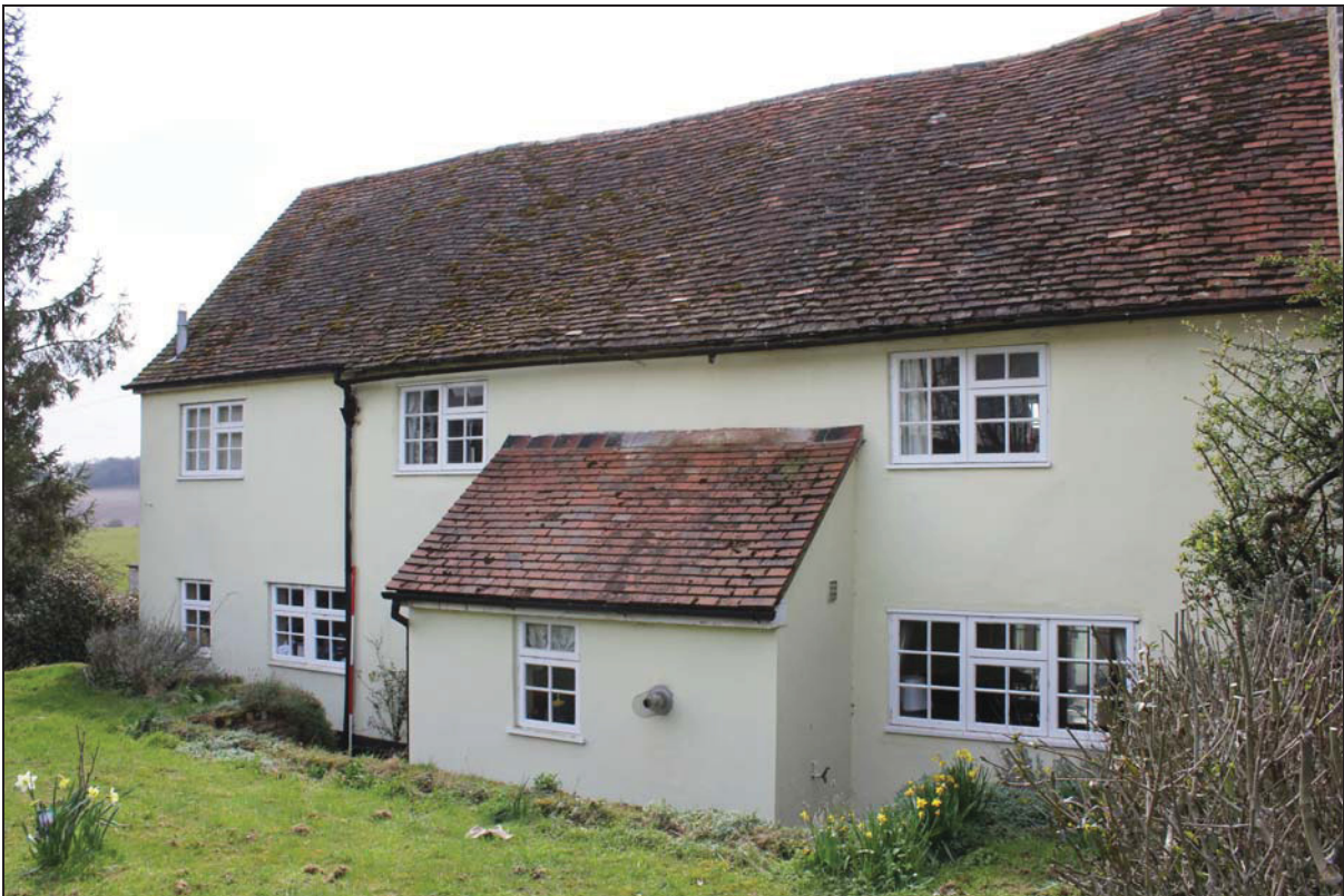
Plate 2 North-east elevation of Lordship Cottage, taken from the north (DP 04)
