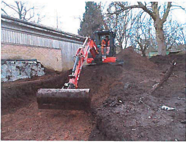
Machine stripping excavation area.
