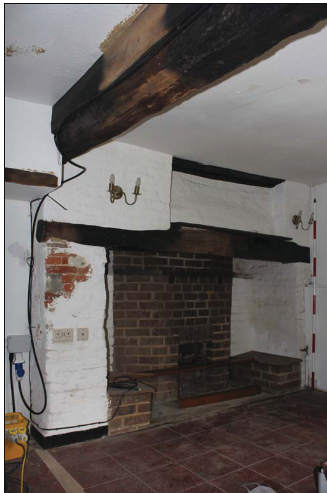
Plate 20 Interior view of GF04, taken from the south-west (DP 052)
