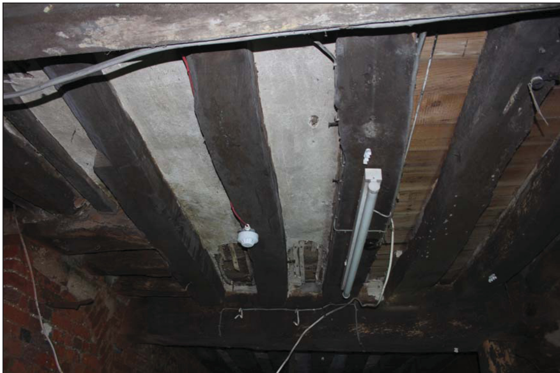
Plate 12 Ceiling joists in the basement, taken from the west (DP 309)
