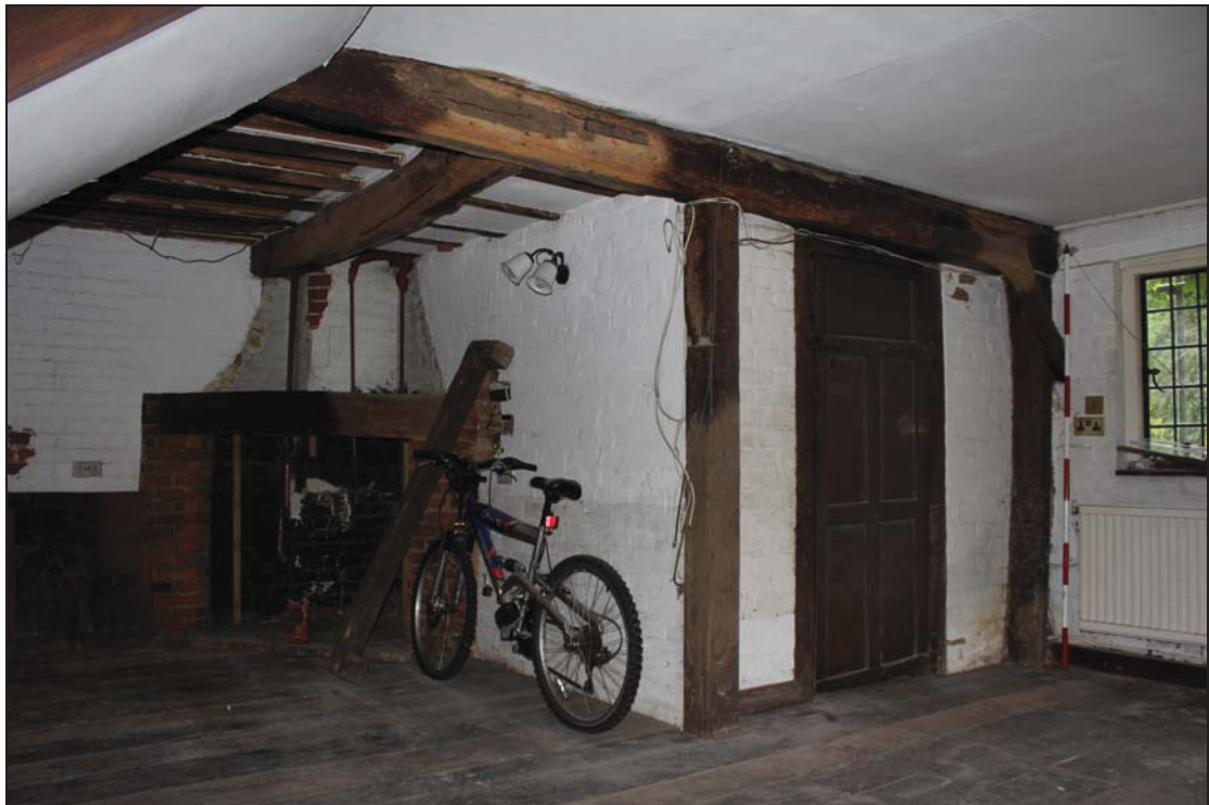
Plate 42 Interior view of GF10, taken from the south-west (DP 099)
