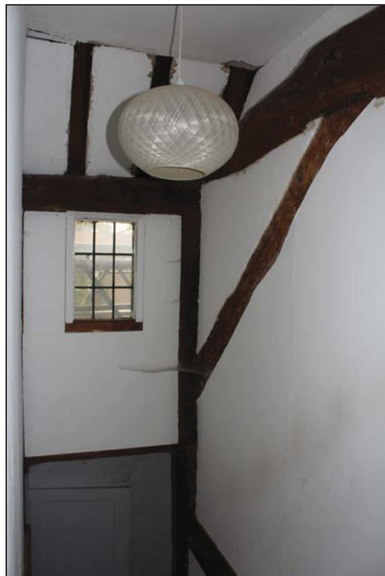
Plate 46 Timber-framing above the stairs in FF15, taken from the east (DP 156)
