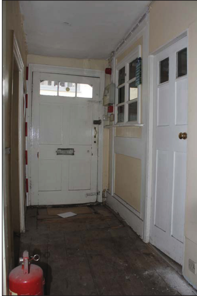
Plate 11 Entrance corridor (GF01), taken from the south (DP 020)
