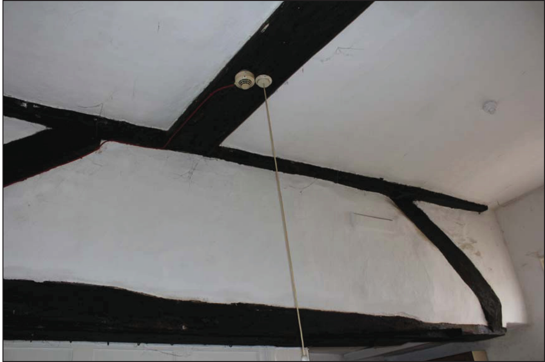
Plate 17 Timber-framing in GF03, taken from the south-east (DP 042)
