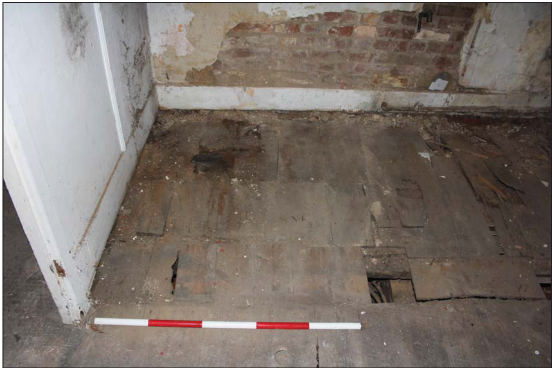
Plate 18 Exposed floorboards in GF03, taken from the south (DP 262)
