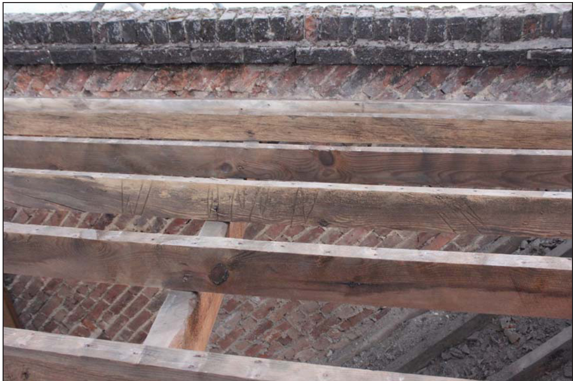
Plate 34 Baltic marks on the rafters of the west front range, taken from the east (DP 236)
