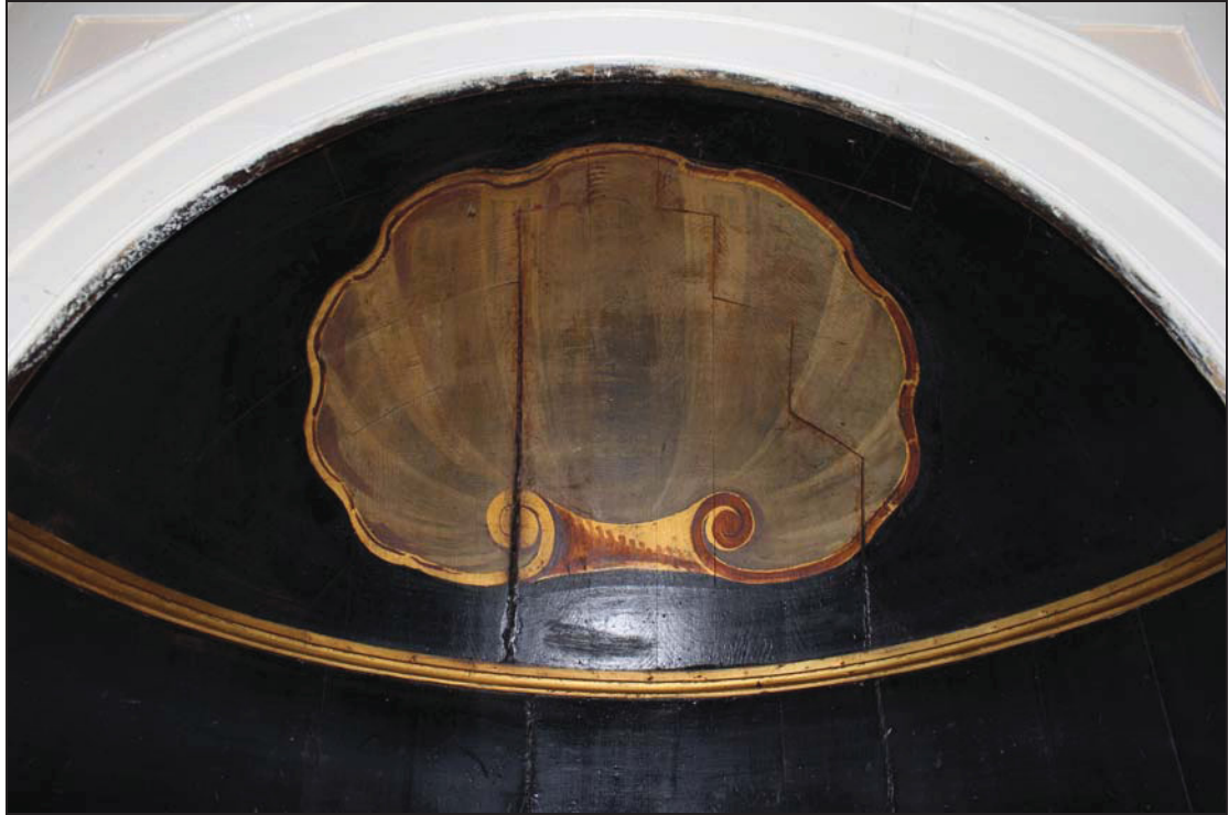
Plate 15 Painted scallop shell detailing in the 18th century cupboard in GF01, taken from the north-west (DP 031)
