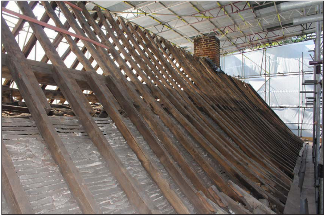
Plate 49 Roof structure over the rear range, taken from the north-west (DP 196)
