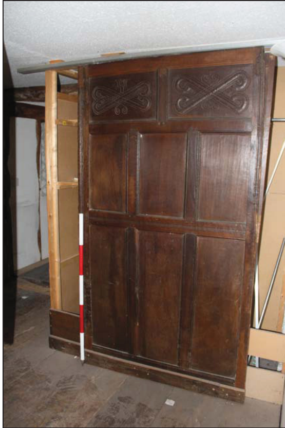
Plate 47 A closet formed with 17 th century panelling in FF11, taken from the south (DP 165)
