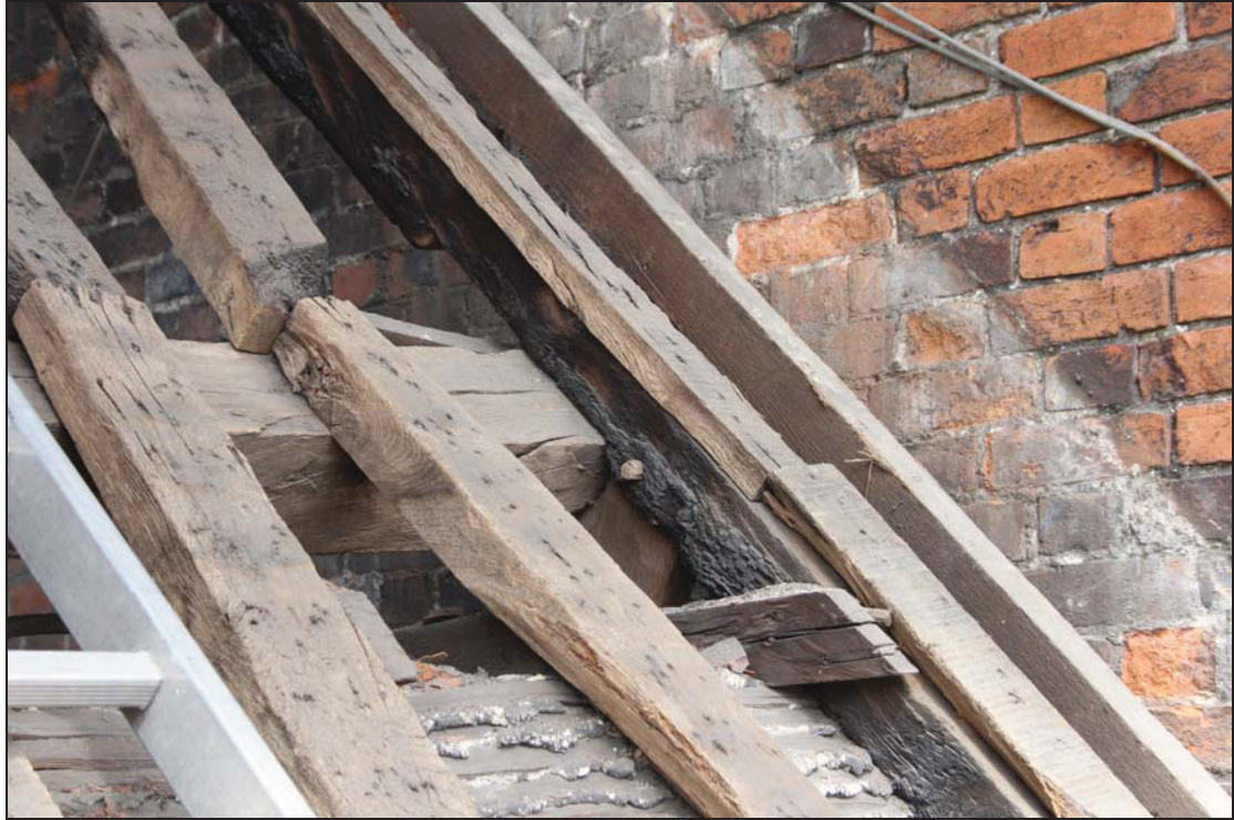
Plate 53 Evidence of smoke-blackening and rafter replacement in the roof of the rear range, taken from the south-east (DP 226)
