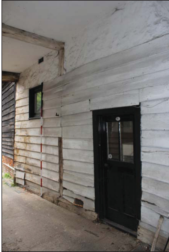
Plate 3 West side of the carriageway, taken from the north-east (DP 012)
