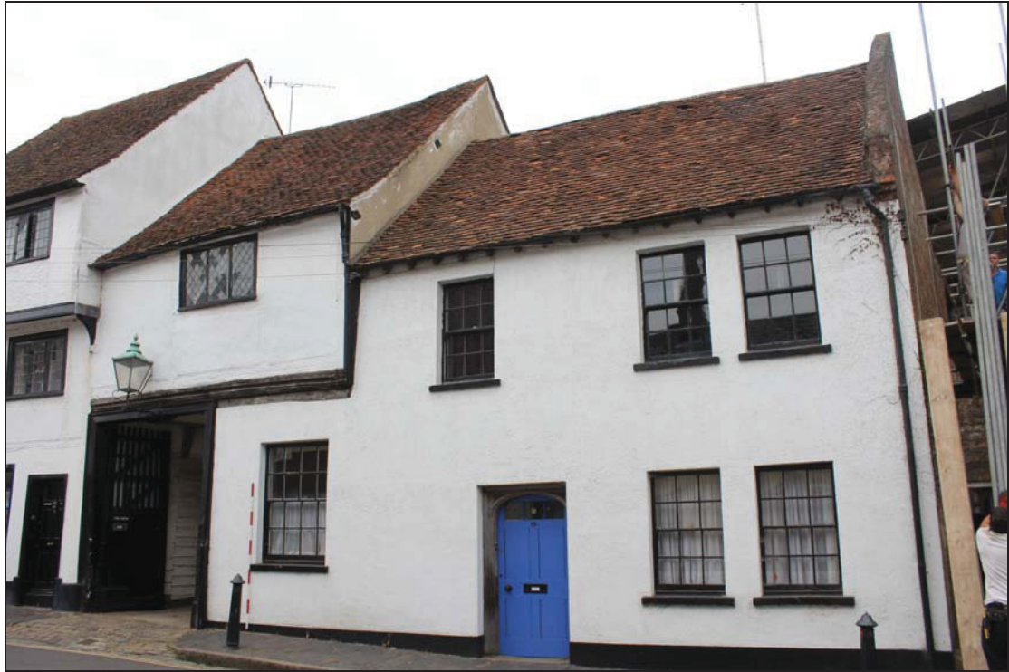
Plate 1 Exterior of No. 15 Fishpool Street, taken from the north (DP 003)
