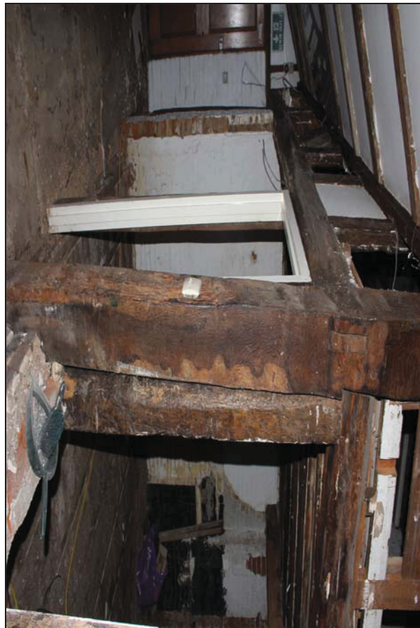
Plate 40 Timber-framing in GF09 comprising the formerly external wall of the rear range, taken from the south-west (DP 295)
