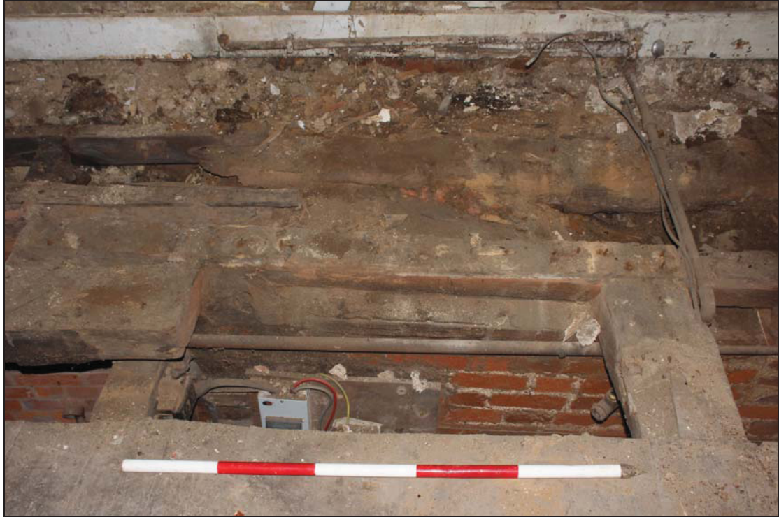
Plate 19 Revealed floor joists in GF03, taken from the south (DP 297)
