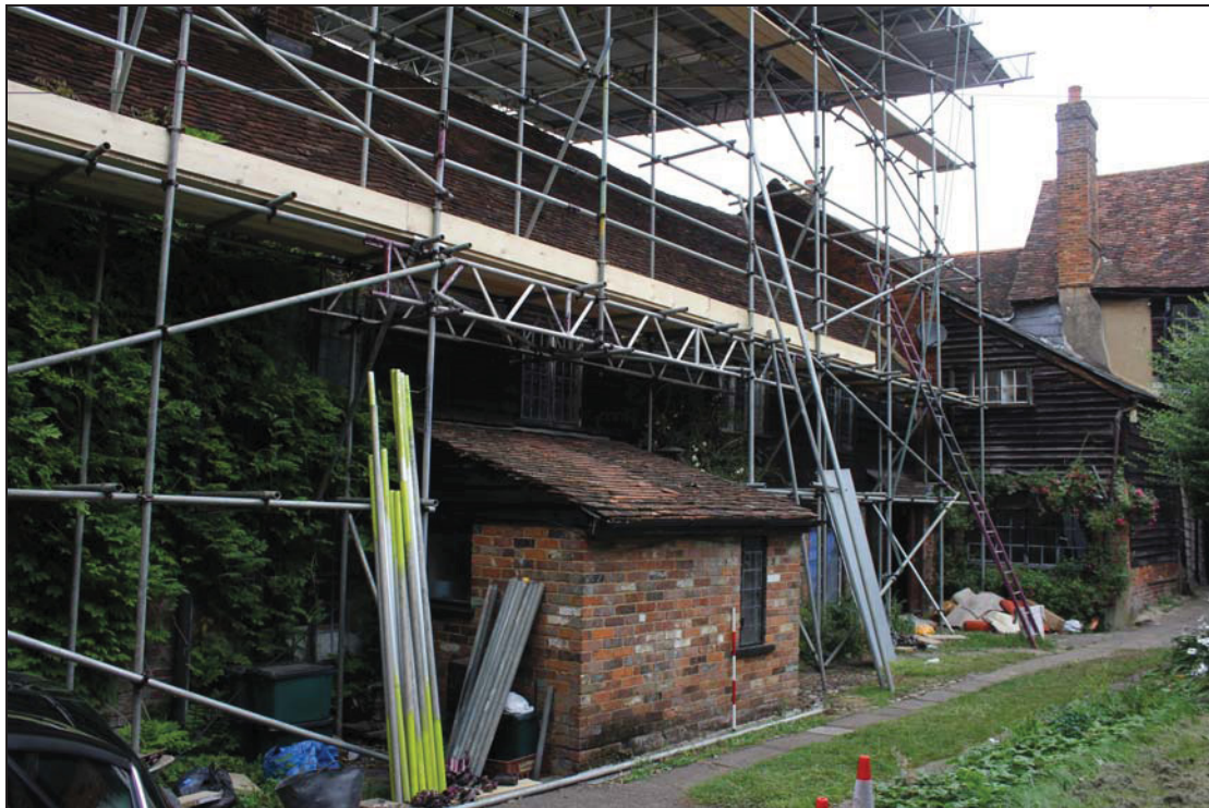
Plate 6 East elevation of the rear range, taken from the south-east (DP 017)
