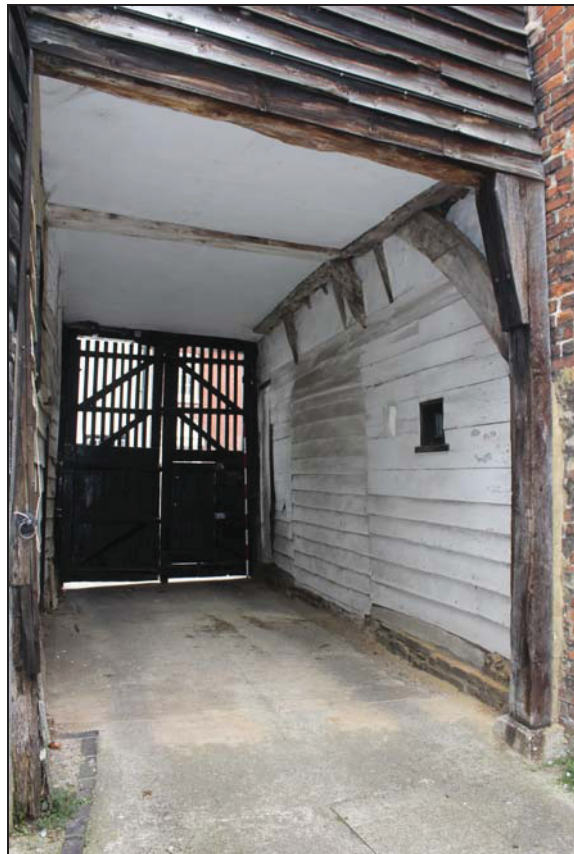
Plate 4 The east side of the carriageway, taken from the south (DP 010)
