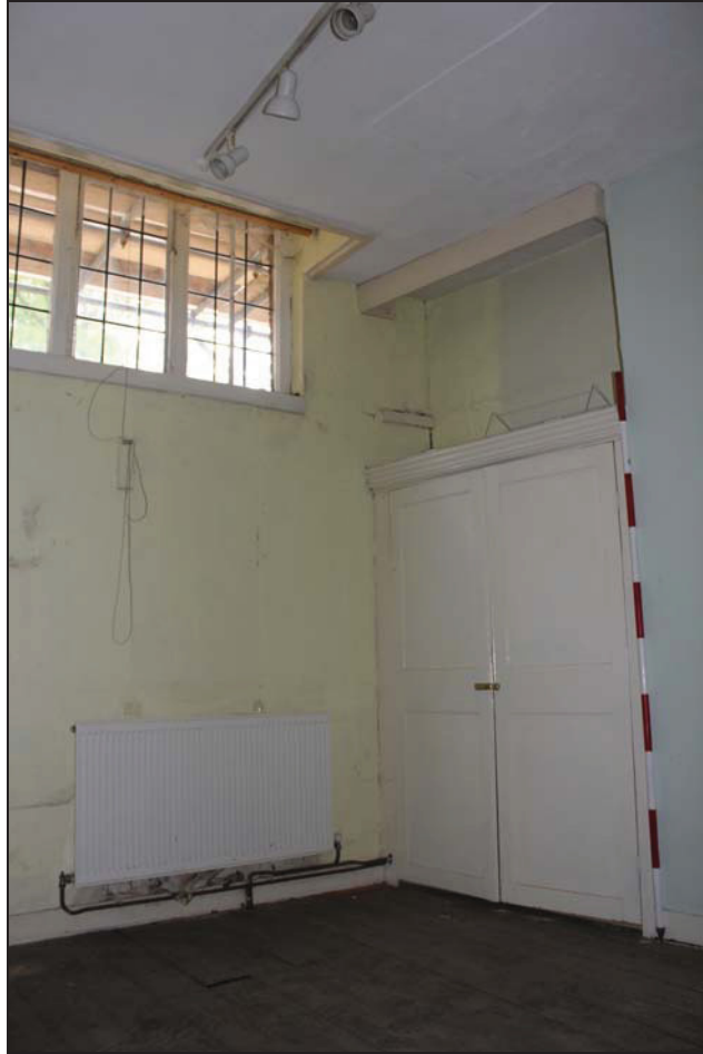
Plate 29 Interior of FF05, taken from the south-east (DP 126)
