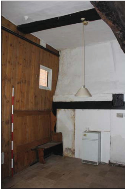
Corbel and bridging joist in GF01, taken from the north.
