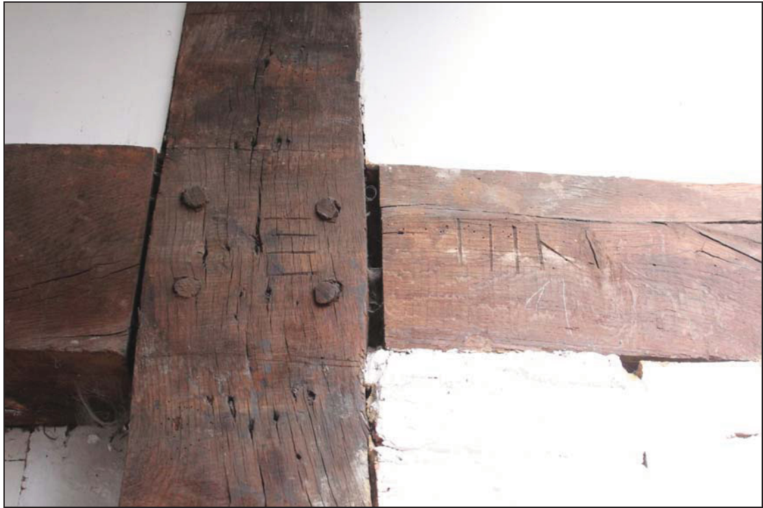
Plate 41 Timber-framing in GF09 with assembly markings, taken from the west (DP 087)
