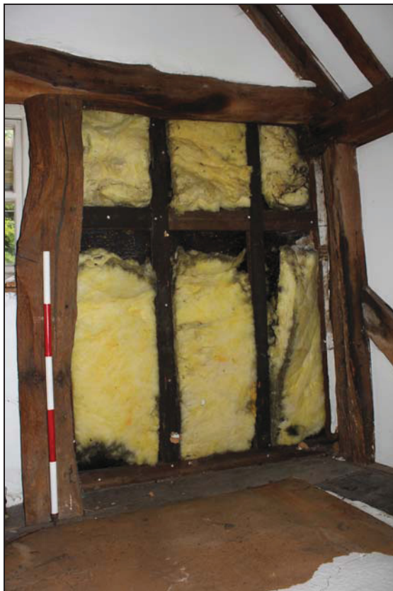
Plate 48 Timber-framing in FF15, taken from the north (DP 158)
