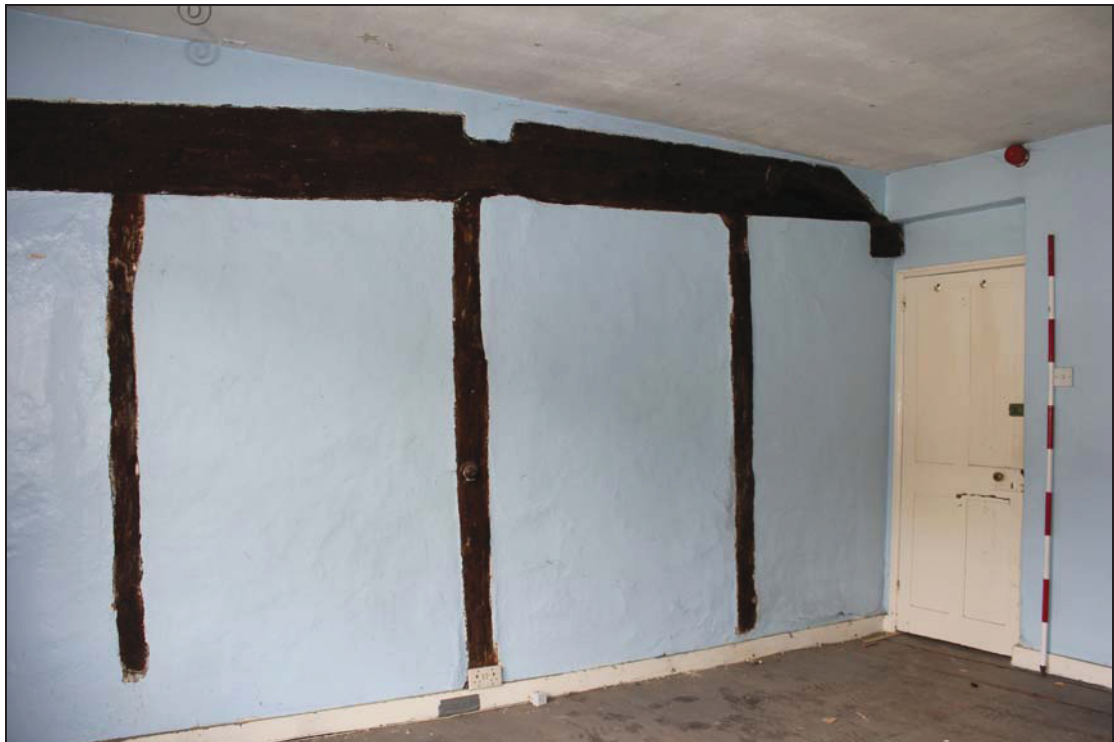
Plate 26 Interior of FF03, with elements of timber-framing including tie-beam and truncated stub of a wall plate above the door, taken from the north-west (DP 128)
