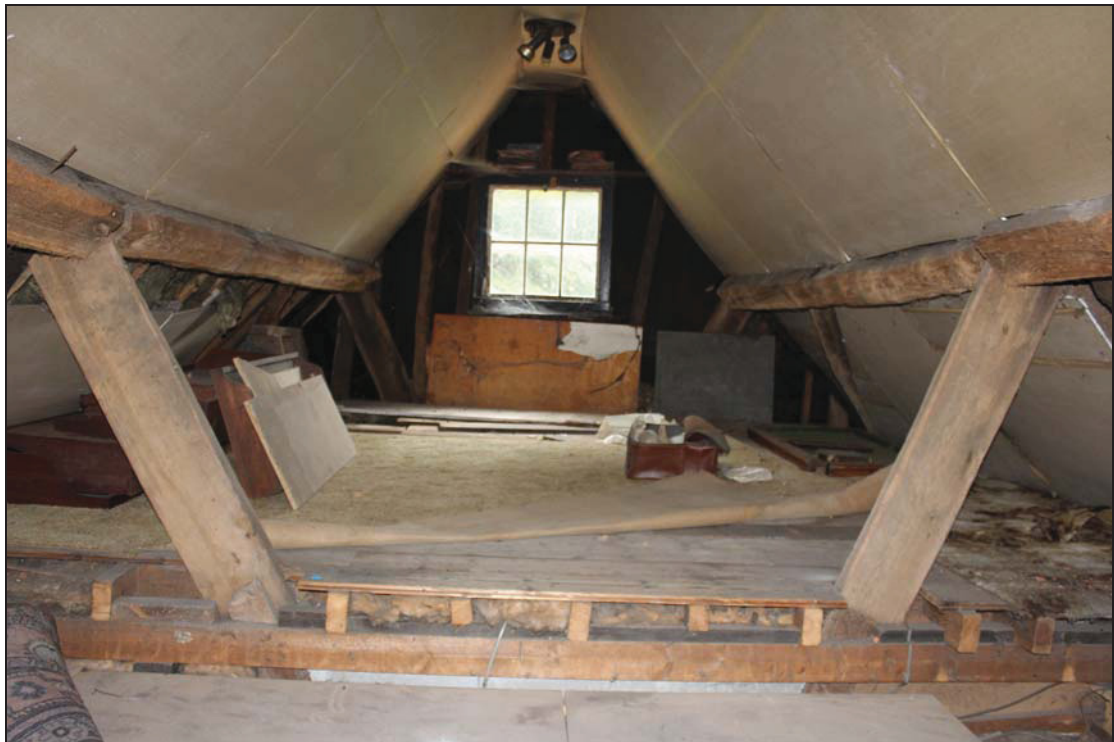
Plate 50 Roof structure over the rear range, taken from the north (DP 174)
