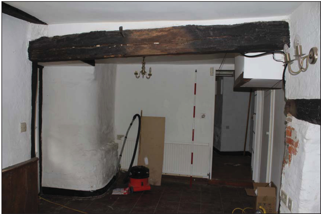
Plate 21 Interior view of GF05, with the bevelled north-east corner of the rear range, taken from the east (DP 059)
