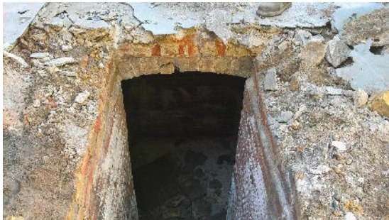
13: Cellar entrance, looking NE
