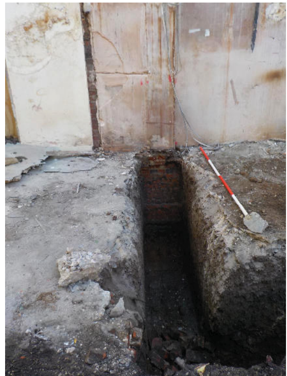
10: Exterior rear footings, looking NW
