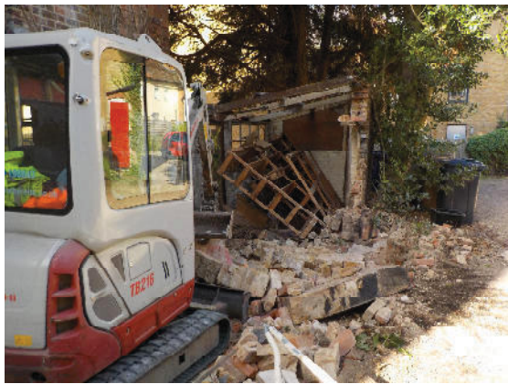
9: Demolition of rear outbuildings, looking NE
