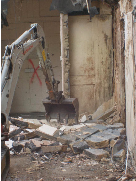
7: Demolition of rear outbuildings, looking SW
