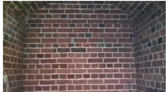
14: Cellar Interior showing English bond brickwork, looking NE
