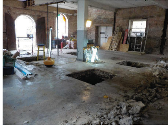
2: Interior view of Footings 1-4 and backfilled service trench, looking N
