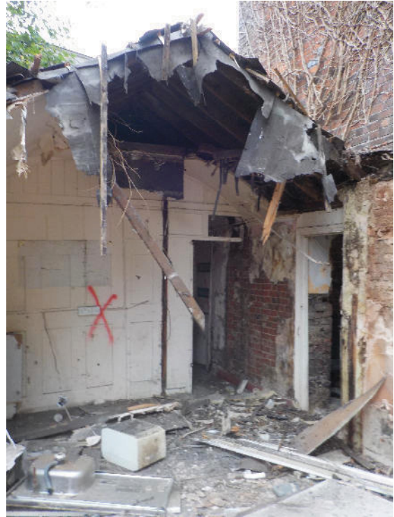
8: Demolition of rear outbuildings, looking SW
