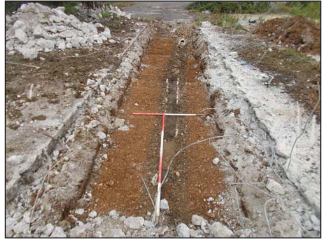
2 View of Trench 2 looking north-west
