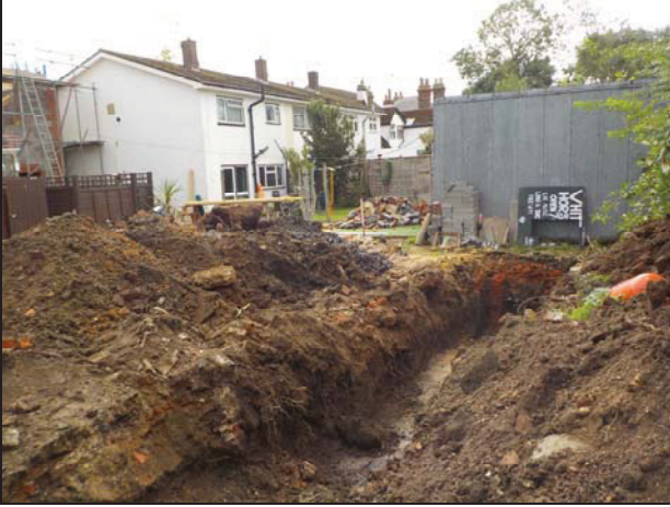
1 View of site looking south-east
