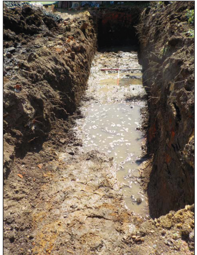
4 View of Trench looking south-west
