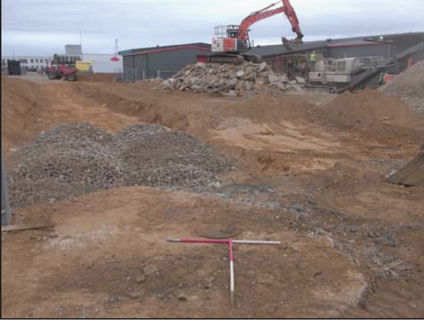
1 View of Site looking south
