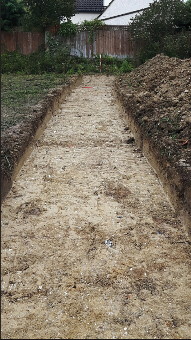
1 View of Trench 1 looking north
