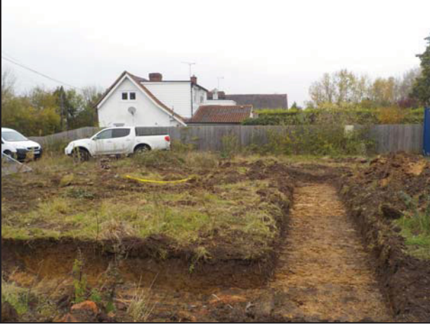
1 View of site looking north
