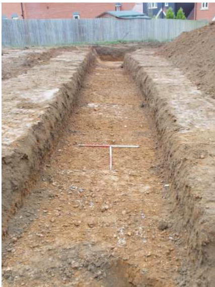
DP 3. Trench 1. Looking north-east.
