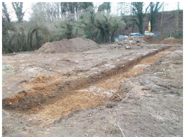
DP 6. Trench 2. Looking south-east.
