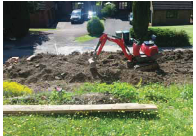
DP 2. View SW across site from adjacent to existing house
