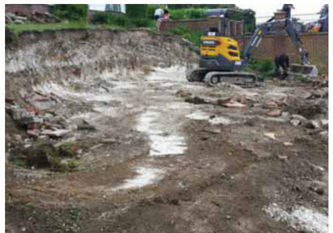
DP 6. View NE across site during ground reduction
