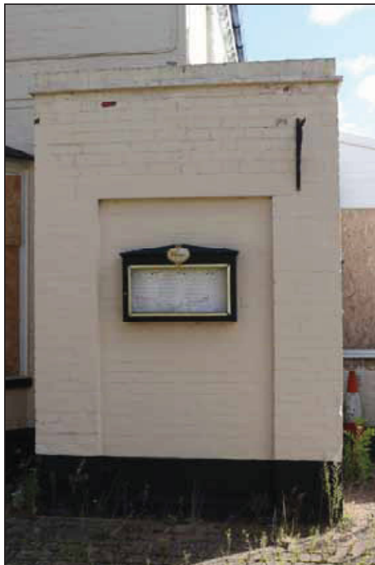
Plate 2 Hotel's secondary entrance porch, taken from the west (DP 032)
