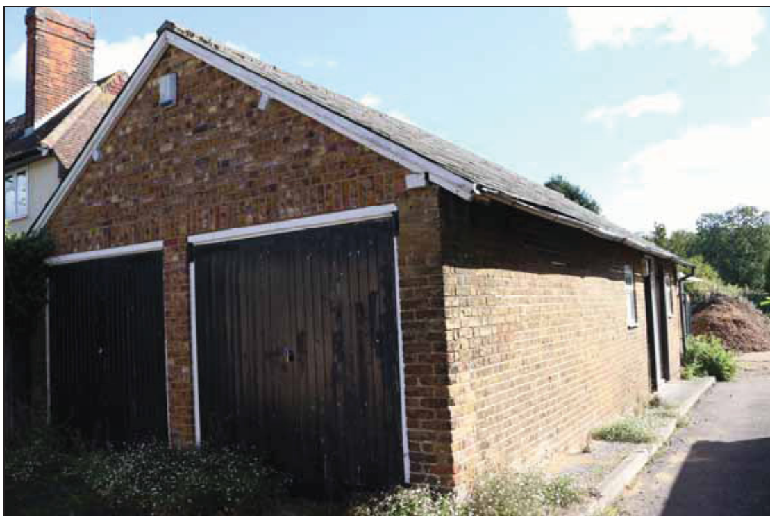
Plate 18 External view of the outbuilding, taken from the south-west (DP 003)
