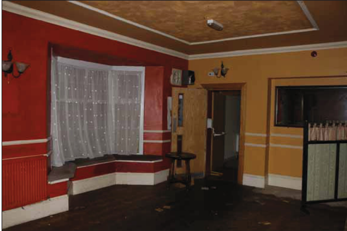
Plate 11 Internal view of the hotel front lounge, taken from the south-east (DP 052)
