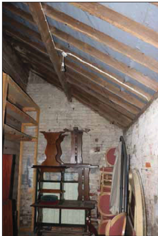
Plate 20 Internal view of the outbuilding, taken from the west (DP 100)
