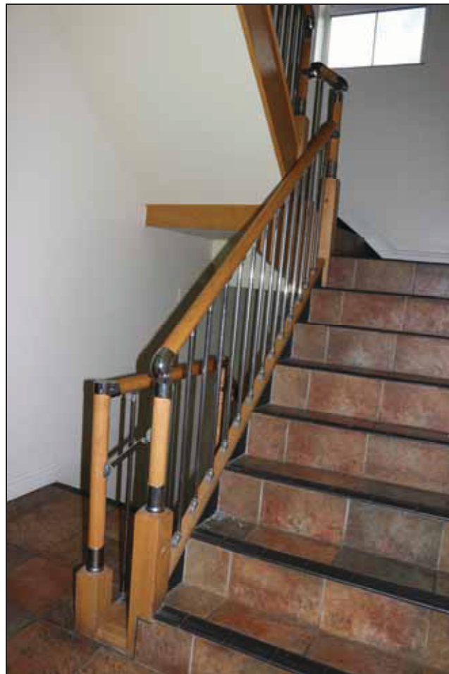
Plate 14 Staircase in the hotel, taken from the south-west (DP_068)
