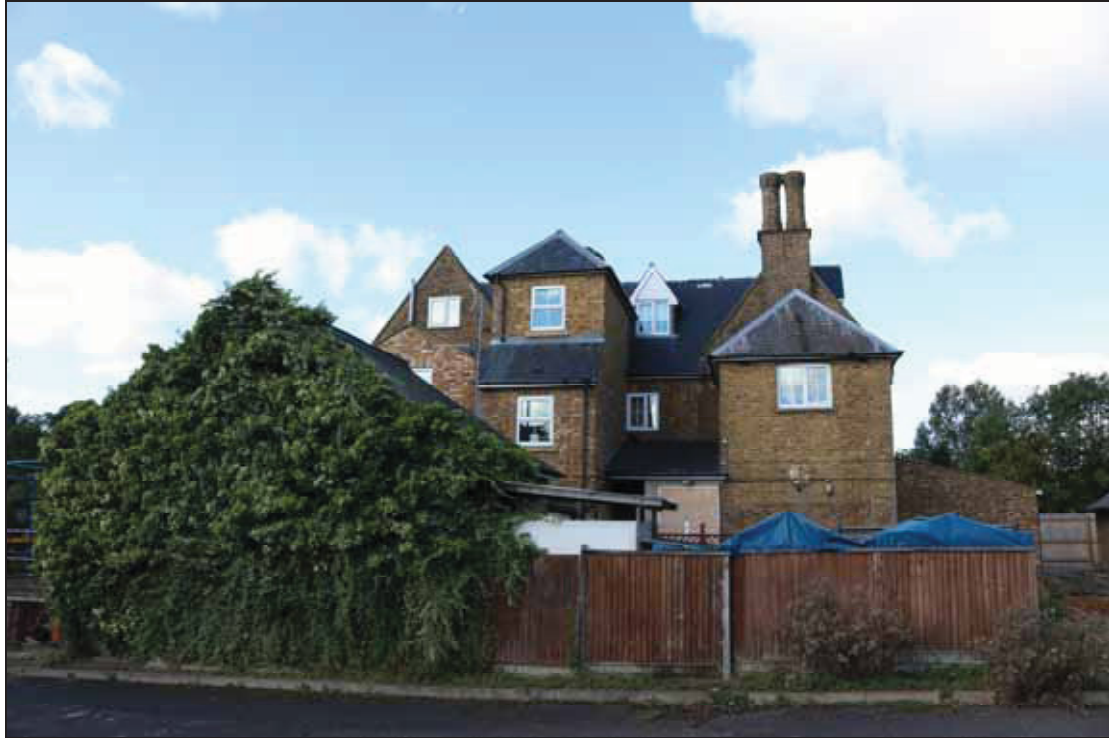
Plate 5 East elevation of the hotel, taken from the east (DP 006)
