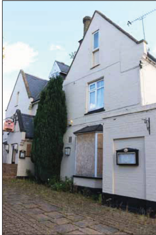
Plate 1 West elevation of the hotel, taken from the south-west (DP 001)
