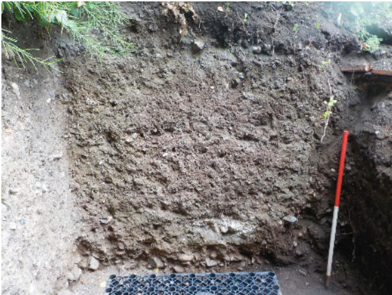
7: West-facing section of soakaway (08/06/2017), looking east (scale = 1m)
