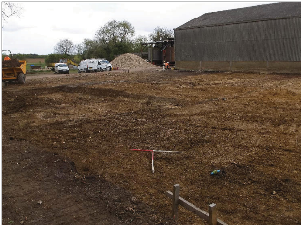
5: Site subsequent to the removal of Structure 2003, looking south-east
