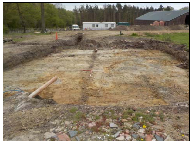
6 View of site looking south
