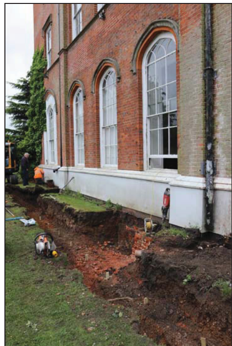
4 Service trench on the north side of the house, looking south-east
