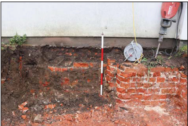
5 Exposed footings on the north elevation of the house, looking south
