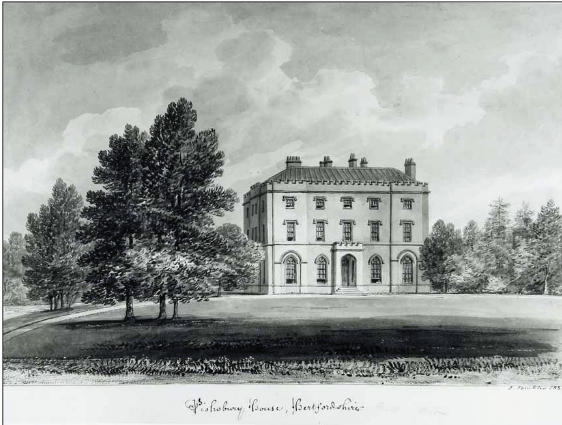
Above: Historical engraving most likely dating to the 19 th century, accessed from HALS.
