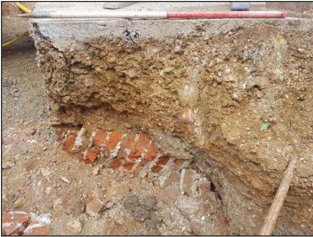
8 Sample section 5 showing section of masonry 1004, looking north-west
