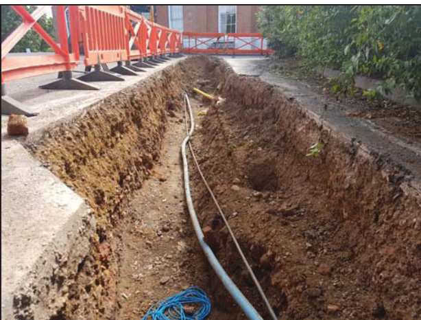
5 Eastern half of the southern service trench, looking east
