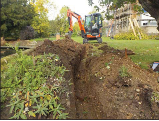
1 Service trenches being excavated
