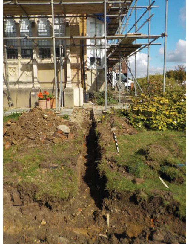
2 Service trench leading to the house
