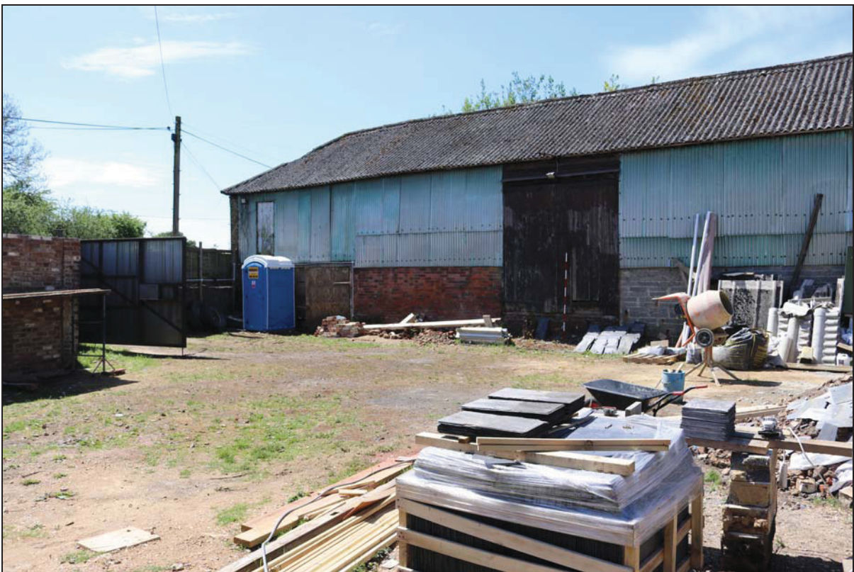
Plate 2 View of the building forming the west side of the farm complex (outside the scope of investigation), taken from the east (DP 29)
