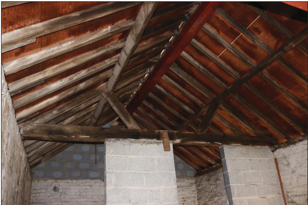
Plate 6 View of Truss 1 (Building 1), taken from the west (DP 37)
