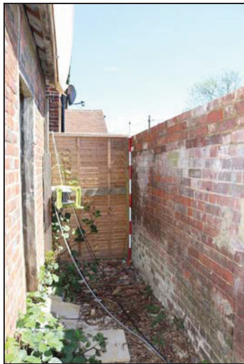
DP 15 North elevation of Building 2 (Unit 1), taken from the west
