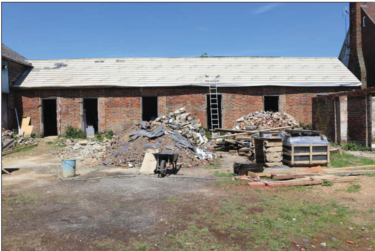
Plate 3 South elevation of Building 1, taken from the south (DP 27)
