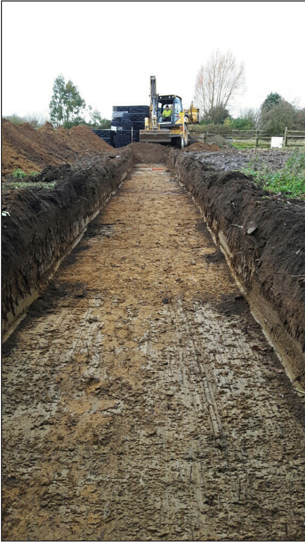
1 Trench 1 looking north-west
