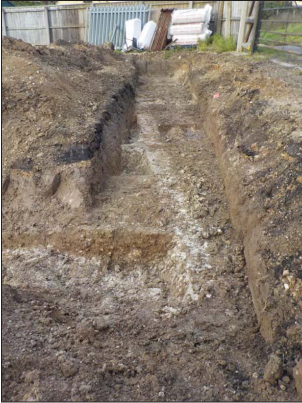
1 View of Trench 1 looking north
