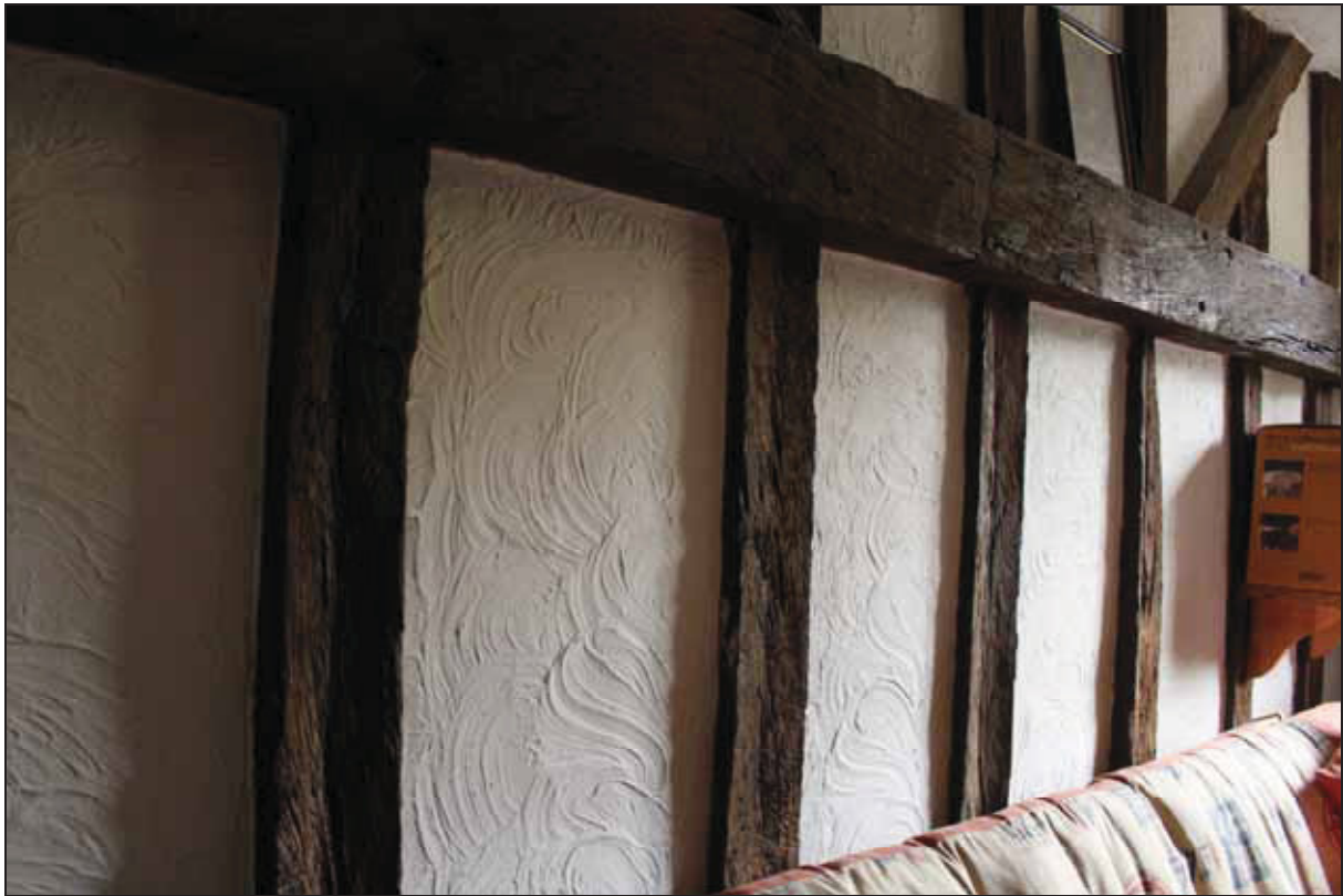
Plate 5 Detail of the studs on the south side of Bay 3 showing characteristic V-shaped depression, taken from the east (DP 17)
