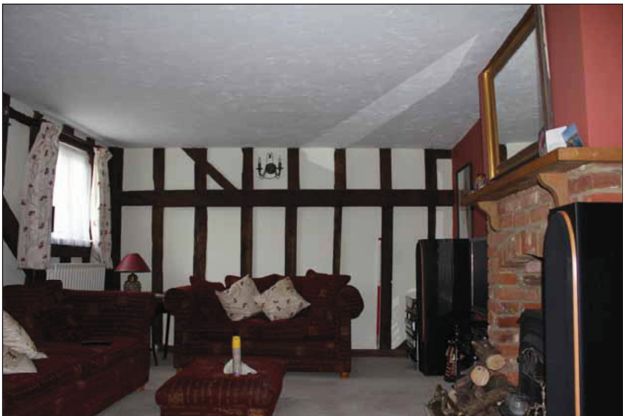
Plate 4 View of Bay 1 (living room) with original framing at the north end, taken from the south-east (DP 23)
