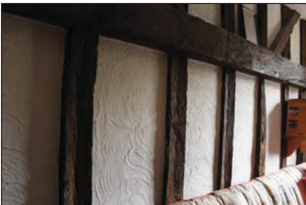
DP 17 Detail of the studs on the south side of Bay 3 showing characteristic V-shaped depression, taken from the east
