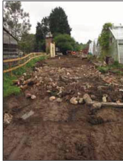
8 Backfill after topsoil strip. Looking northeast
