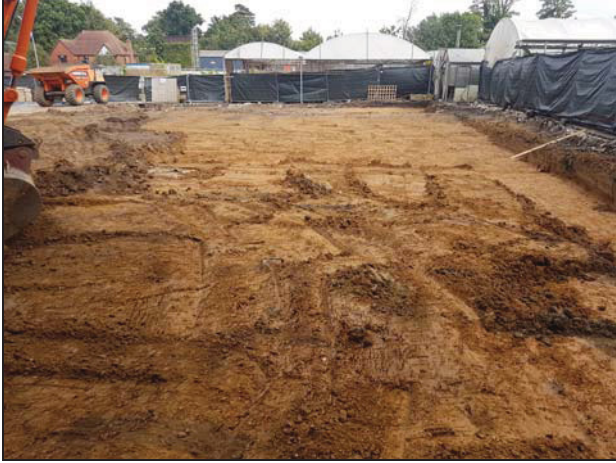
1 View of site after removal of topsoil
