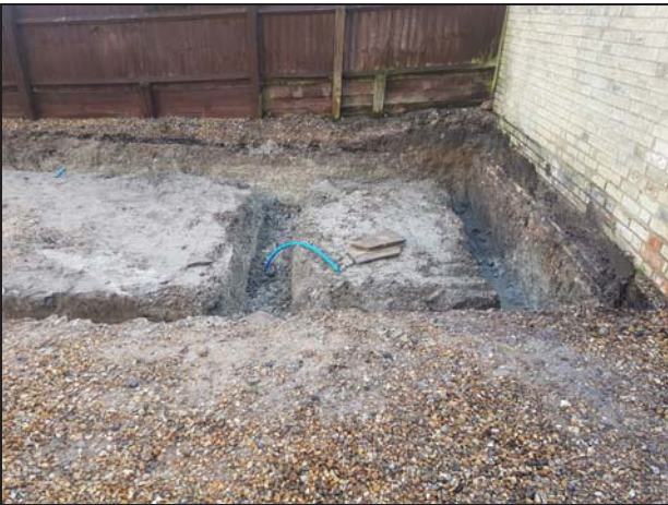
3 View of footings looking north-east
