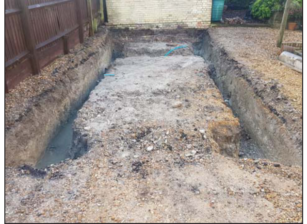
2 View of footings looking south-east
