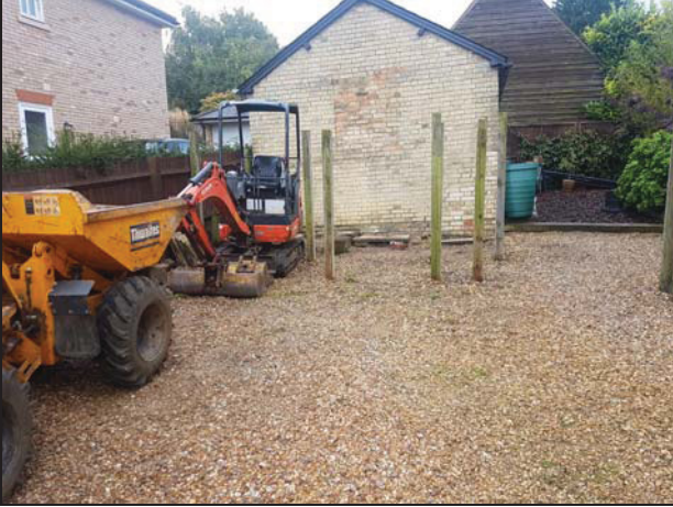
1 View of the site before removal of gravel and tarmac
