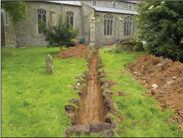
1 General view of northern excavations looking south-west
