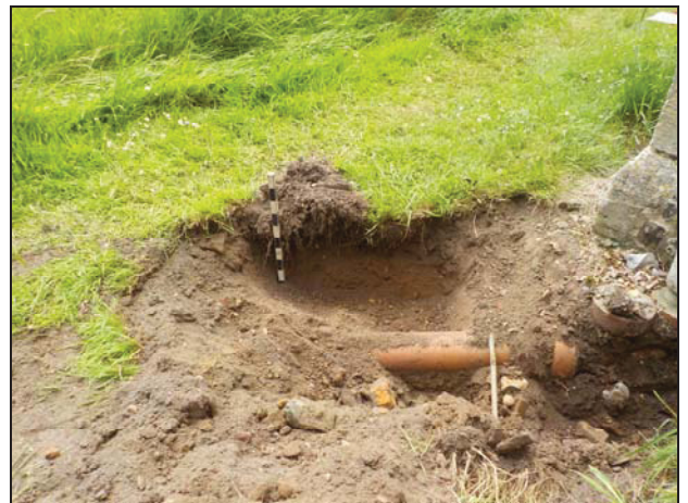
6 Sample Section 5 looking south-west
