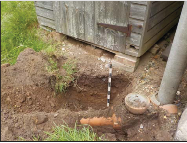
7 Sample Section 6 looking north-west
