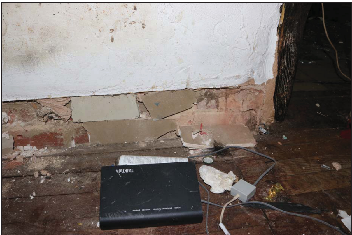
Plate 8 Detail of the internal partition between Rooms GF03 and GF04 showing Fletton brick, taken from the west (DP 22)
