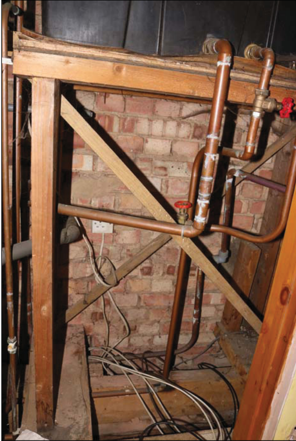
Plate 11 East end of Room SF02 showing Fletton brickwork in the gable, taken from the west (DP 37)
