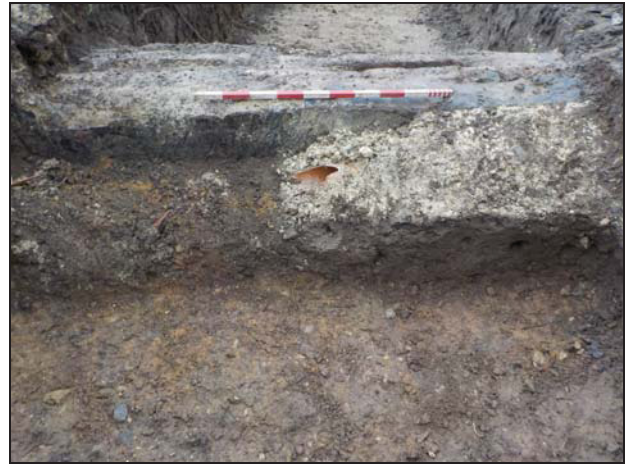
22 Modern wall with plastic pipe encased in concrete in Trench 3
