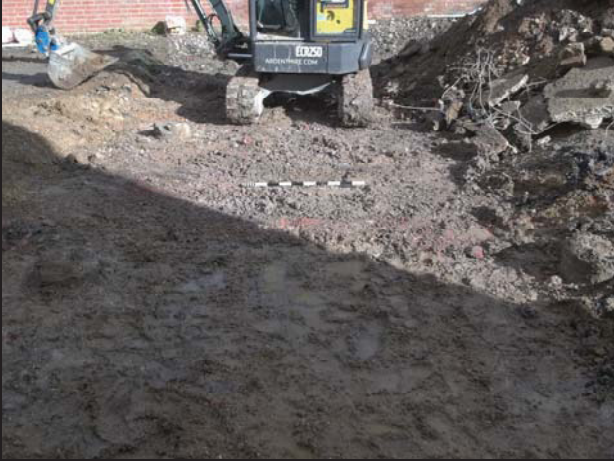
1 General view of site looking north
