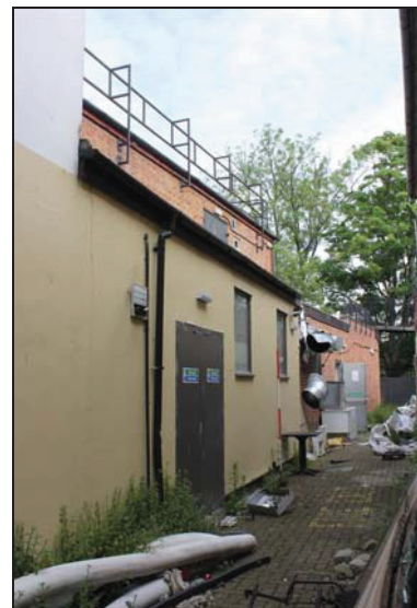
DP 12 East elevation of the rear ranges, taken from the south-east
