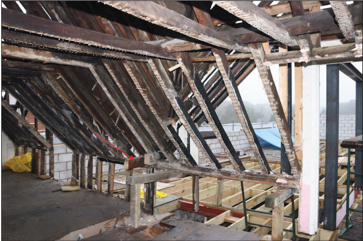
Plate 19 North roof pitch of Bays 3 and 4 (SF01) showing junction between the two with truncated adjacent trusses (indicated), taken from the south-east (DP 140)
