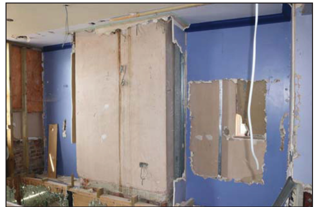
DP 100 North wall of Room SF03 (north-east range) showing surviving timber infilled with brickwork, taken from the south
