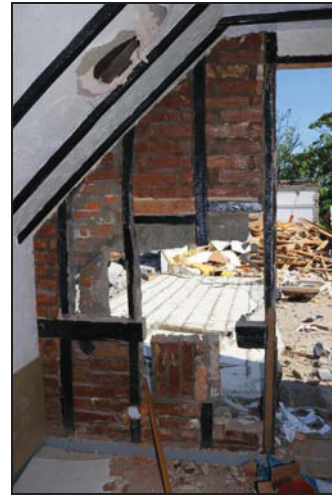
DP 100 North wall of Room SF03 (north-east range) showing surviving timber infilled with brickwork, taken from the south
