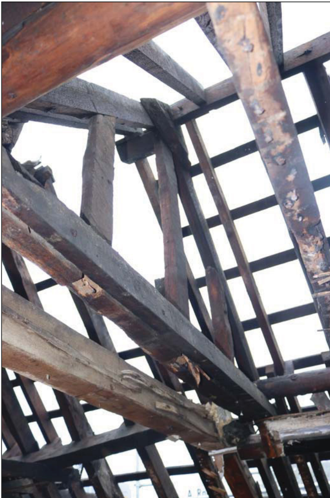
Plate 19 North roof pitch of Bays 3 and 4 (SF01) showing junction between the two with truncated adjacent trusses (indicated), taken from the south-east (DP 140)
