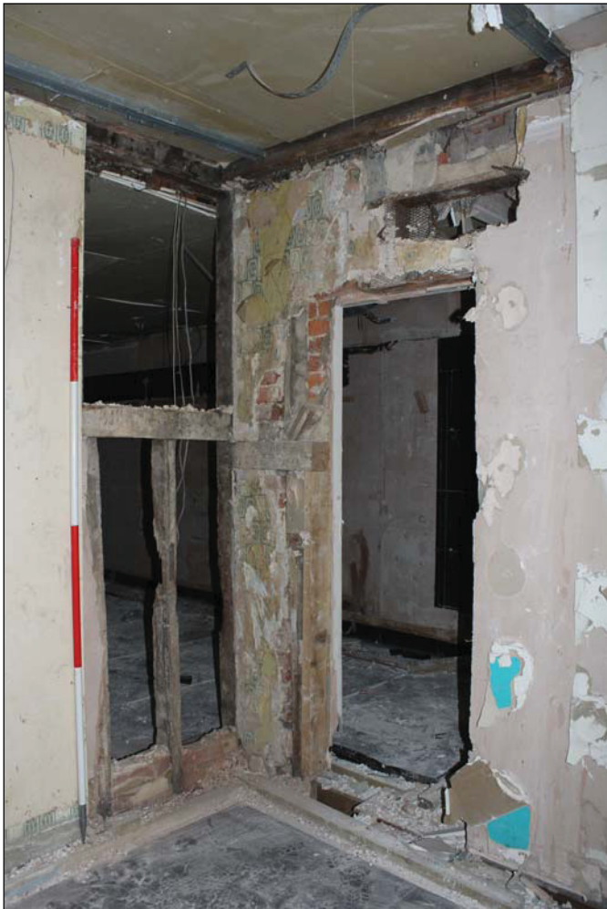
Plate 13 FF04 (north-west range) showing much disturbed fabric including brick and timber and the outline of former chimney flue, taken from the south-east (DP 63)
