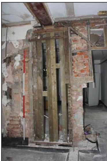
DP 71 Detail of the east side of FF03 (north-east range) showing fragmentary survival of timber framing with much later replacement, taken from the west
