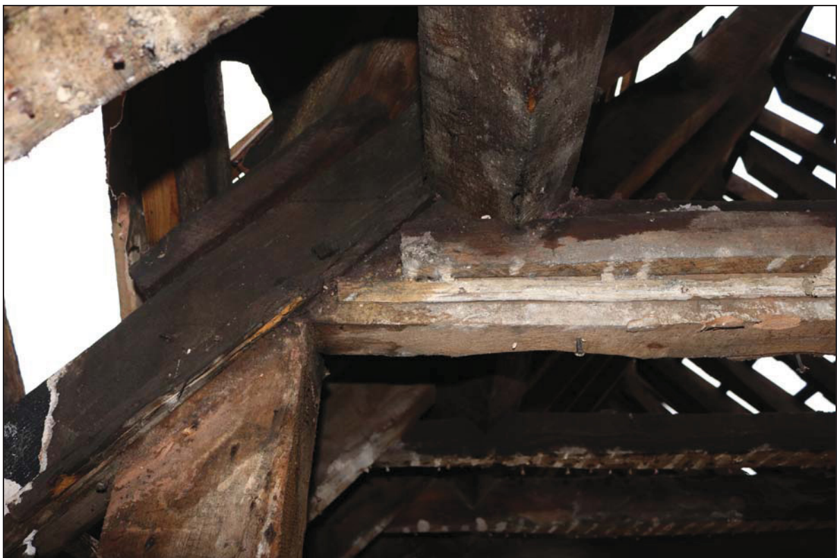
Plate 18 North end of Truss 2 showing collar pegged to the principal rafter and clasping the purlin, taken from the west (DP 144)
