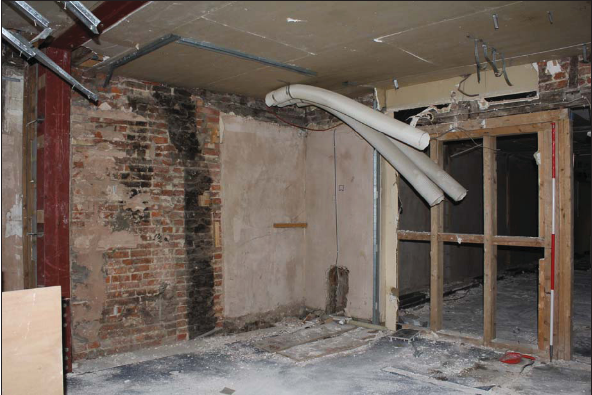
Plate 13 FF04 (north-west range) showing much disturbed fabric including brick and timber and the outline of former chimney flue, taken from the south-east (DP 63)
