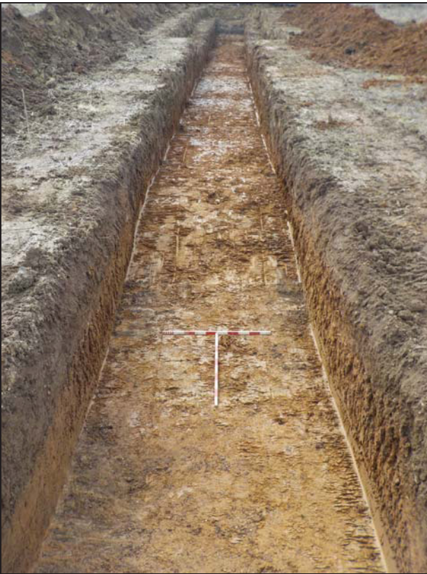
36 Trench 11 looking south-west
